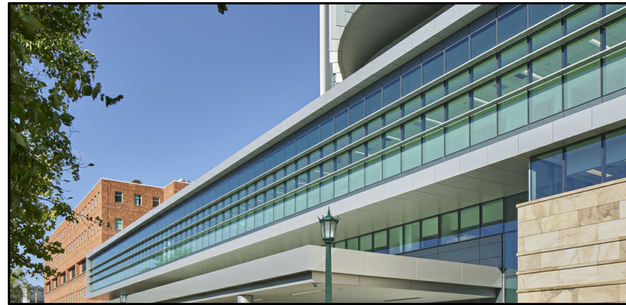
UNIVERSITY OF VIRGINIA HOSPITAL EXPANSION, VA
