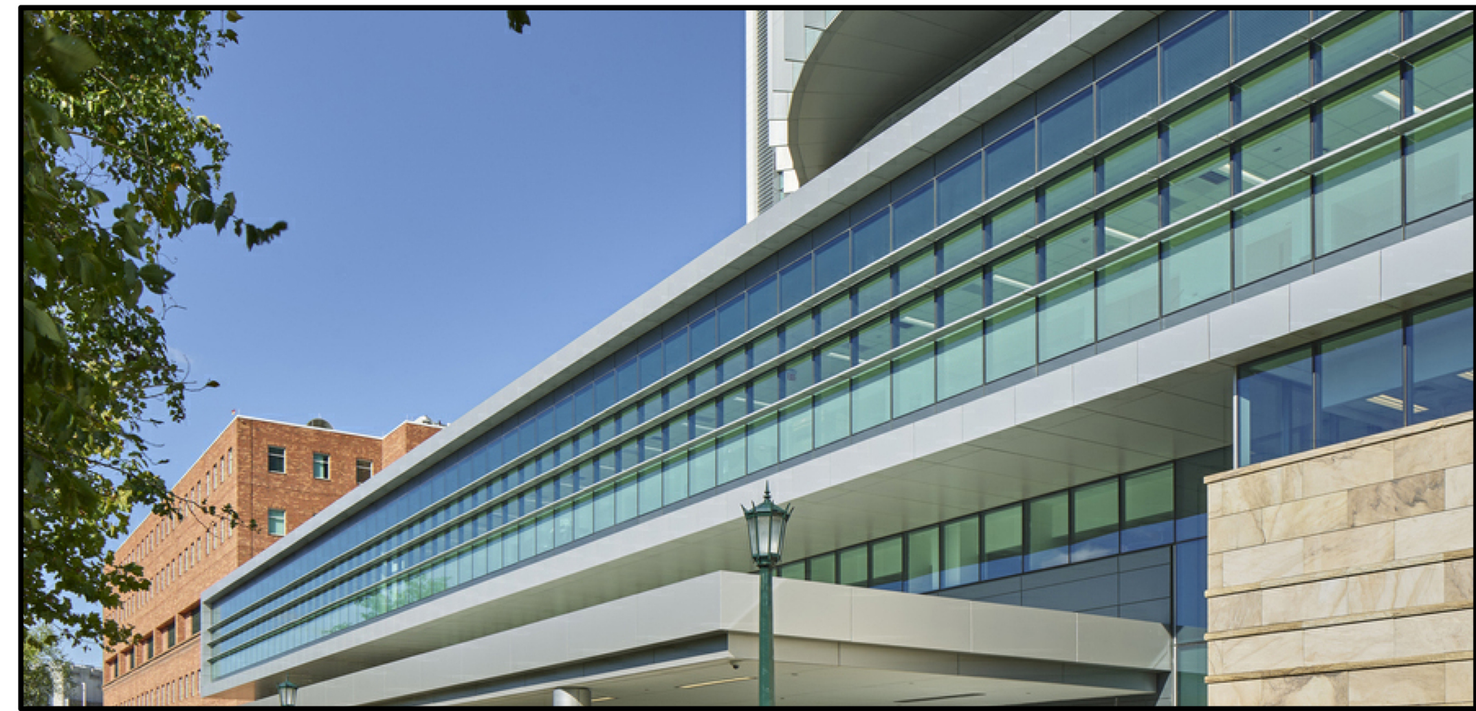
UNIVERSITY OF VIRGINIA HOSPITAL EXPANSION, VA
