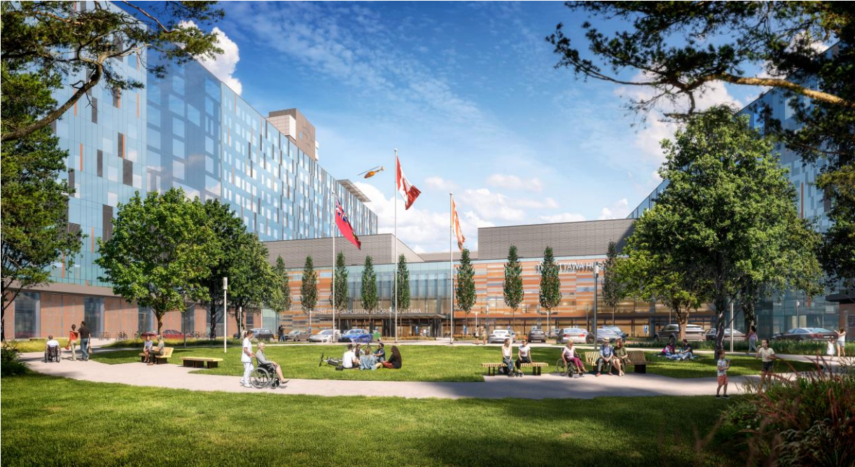
Figure 3.3.1-1: Hospital entry plaza
