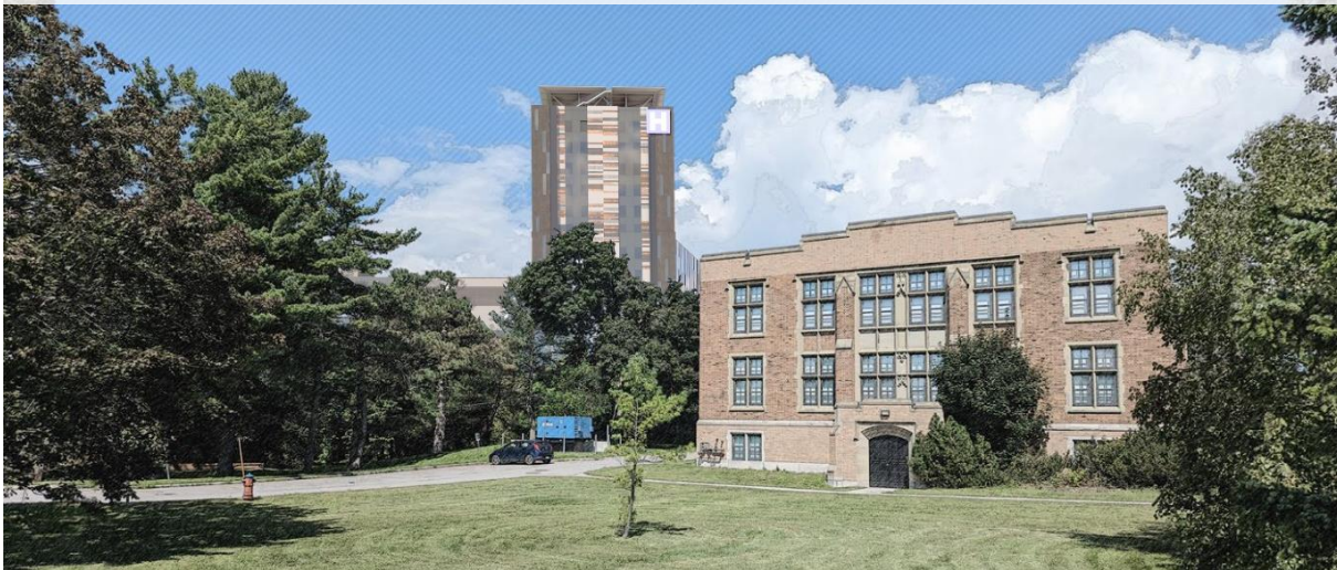
View toward the Saunders Building from Maple Drive
