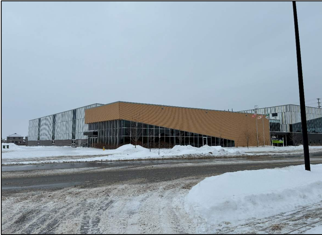
Photograph 7: View looking west at the subject building.
