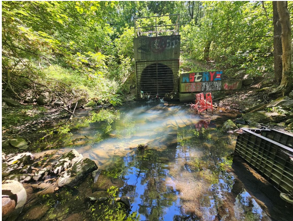
Photo 3: Stormwater Sewer and Large Pool of Stillwater Creek
