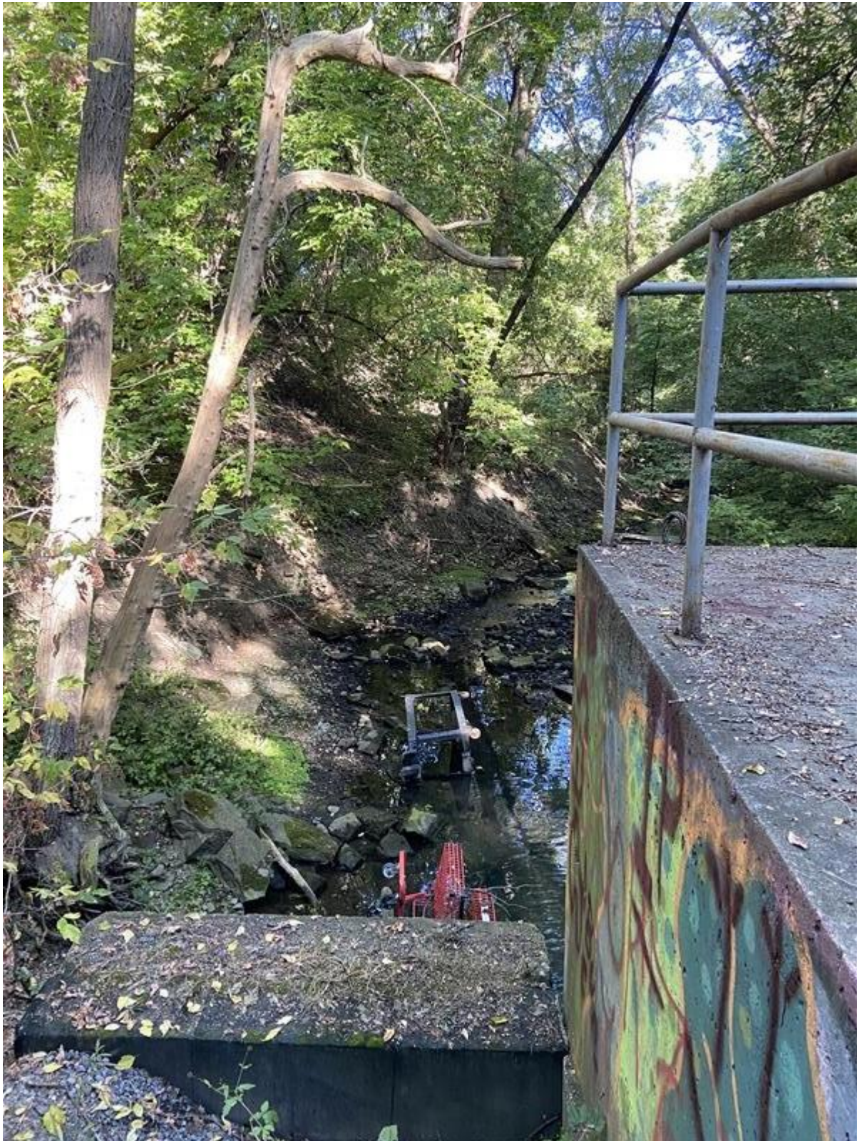
Photo 1: Looking North from the Location of Concrete Culvert – August 15, 2025
