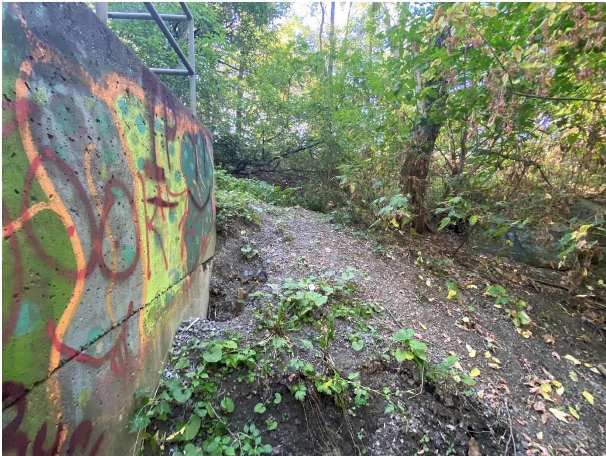
Photo 2: Looking South from the Location of Concrete Culvert – August 15, 2025
