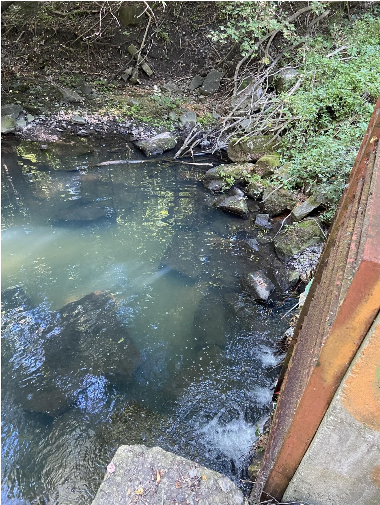
Photo 3: Looking down to the Culvert Outlet – August 15, 2025
