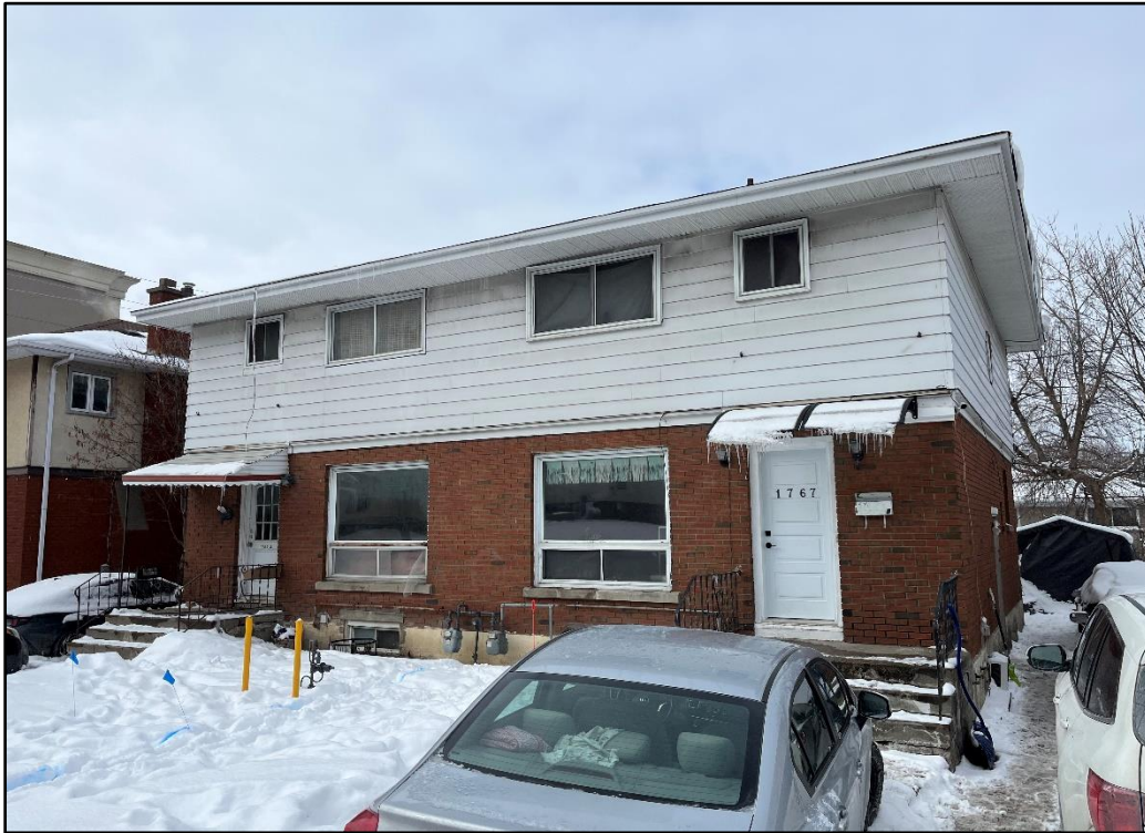
Photograph 1: View looking north at 1767 and 1769 Baseline Road.
