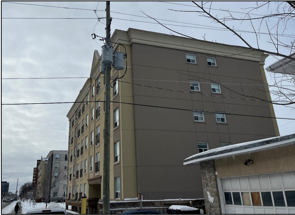
Photograph 7: View looking west at neighbouring residential apartment buildings.
