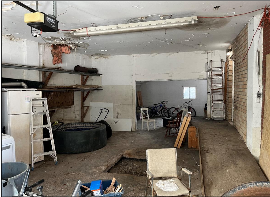
Photograph 5: Representative photo of the garage at 1773 Baseline Road.
