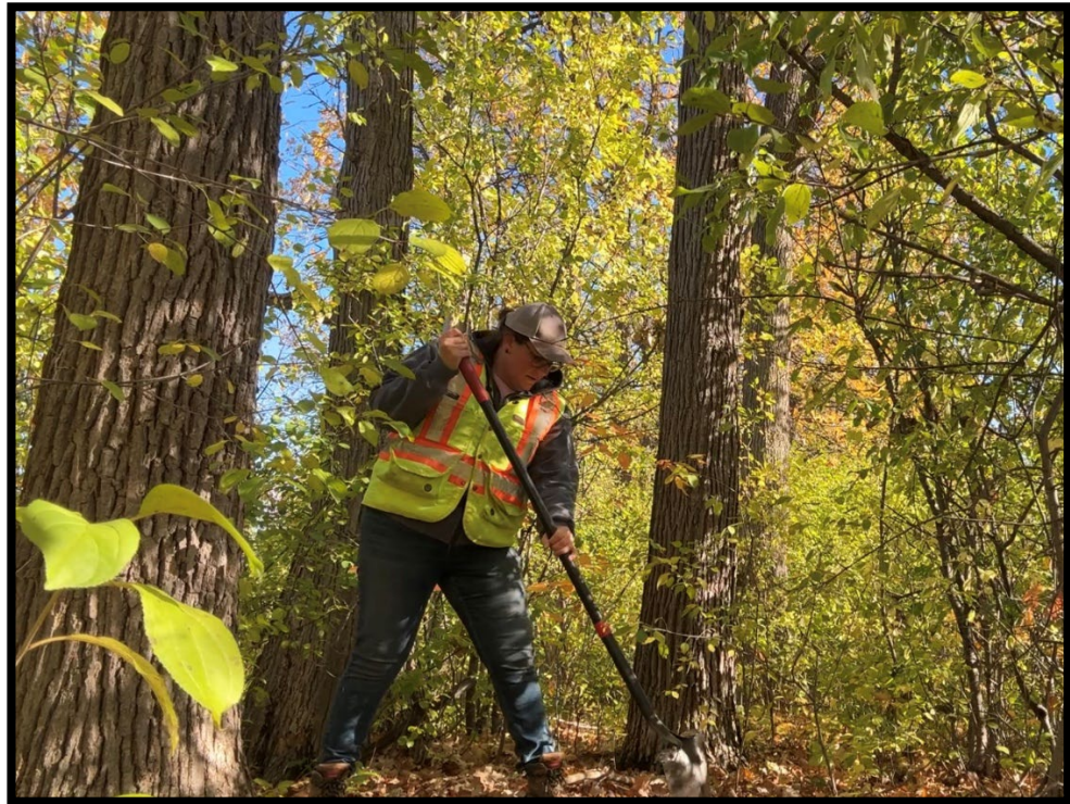
Figure 12: Test pitting in progress (MH1434-D029).
