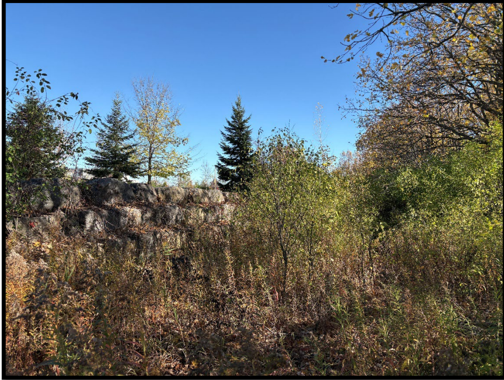
Figure 7: Stone faced berm along northwestern side of study area (MH1434-D024).
