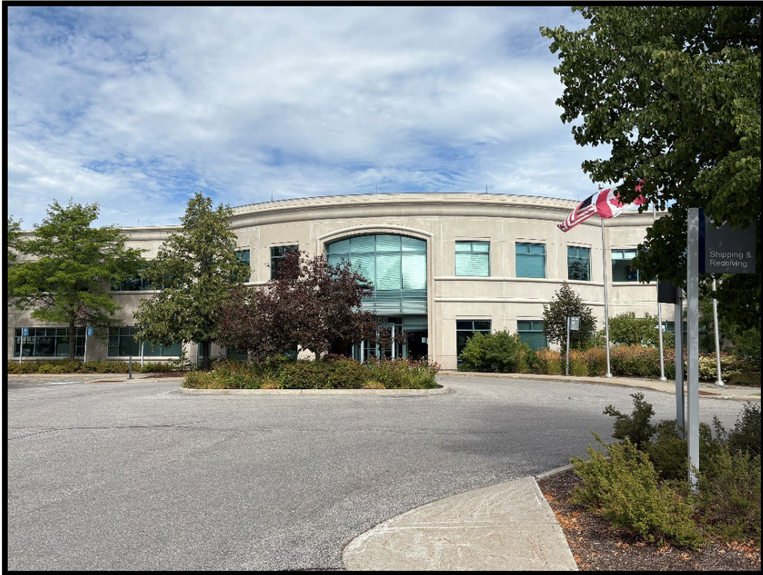
Figure 1: Front entrance of 2000 Innovation Drive (MH1415-D024).
