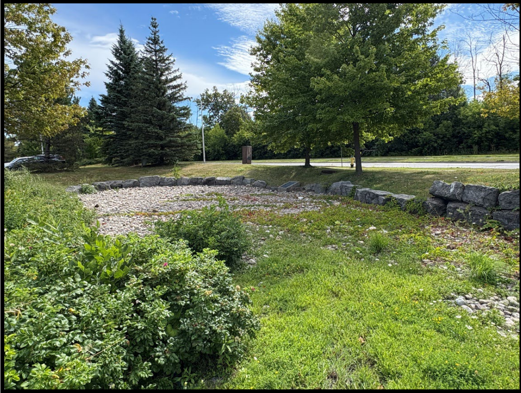
Figure 17: Example of landscaping, with buried utility (MH1415-D014).
