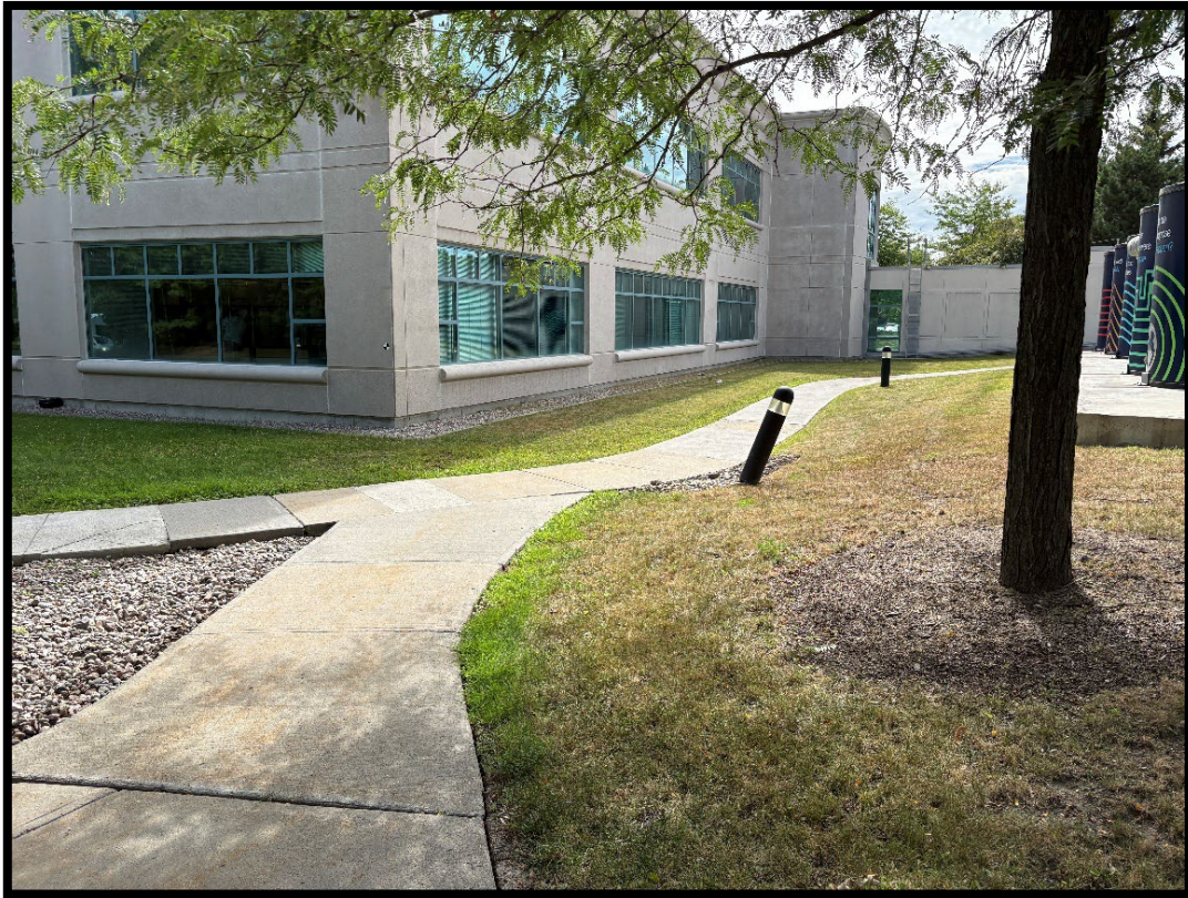
Figure 35: Example of walkways around the buildings to the north (MH1415-D093).
