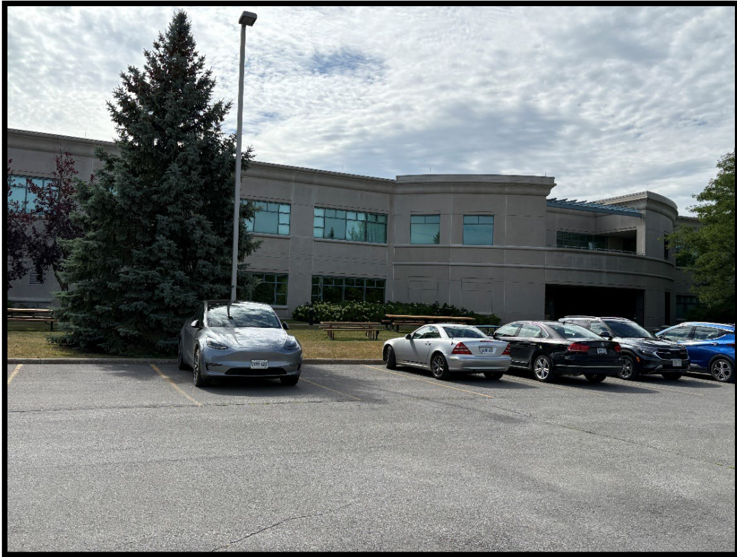
Figure 3: Rear entrance of 2000 Innovation Drive (MH1415-D105).
