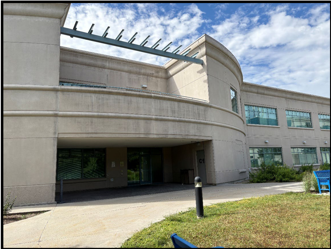
Figure 2: Rear entrance of 3000 Innovation Drive (MH1415-D089).
