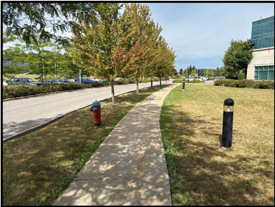
Figure 28: Example of multiple buried utilities (MH1415-D124).
