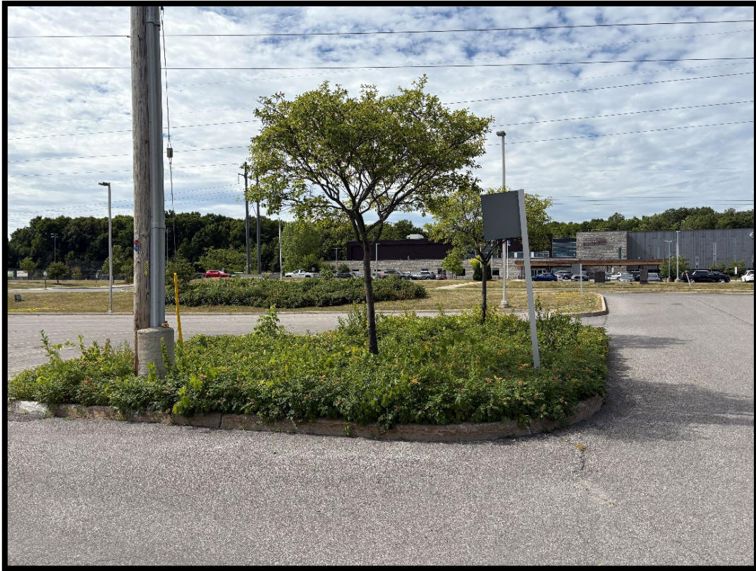
Figure 29: Example of buried utilities within landscaping features in the parking lot (MH1415-D131).
