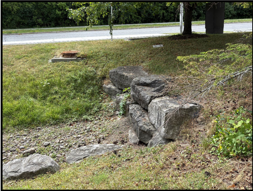
Figure 25: Example of multiple buried utilities within landscaping (MH1415-D026).
