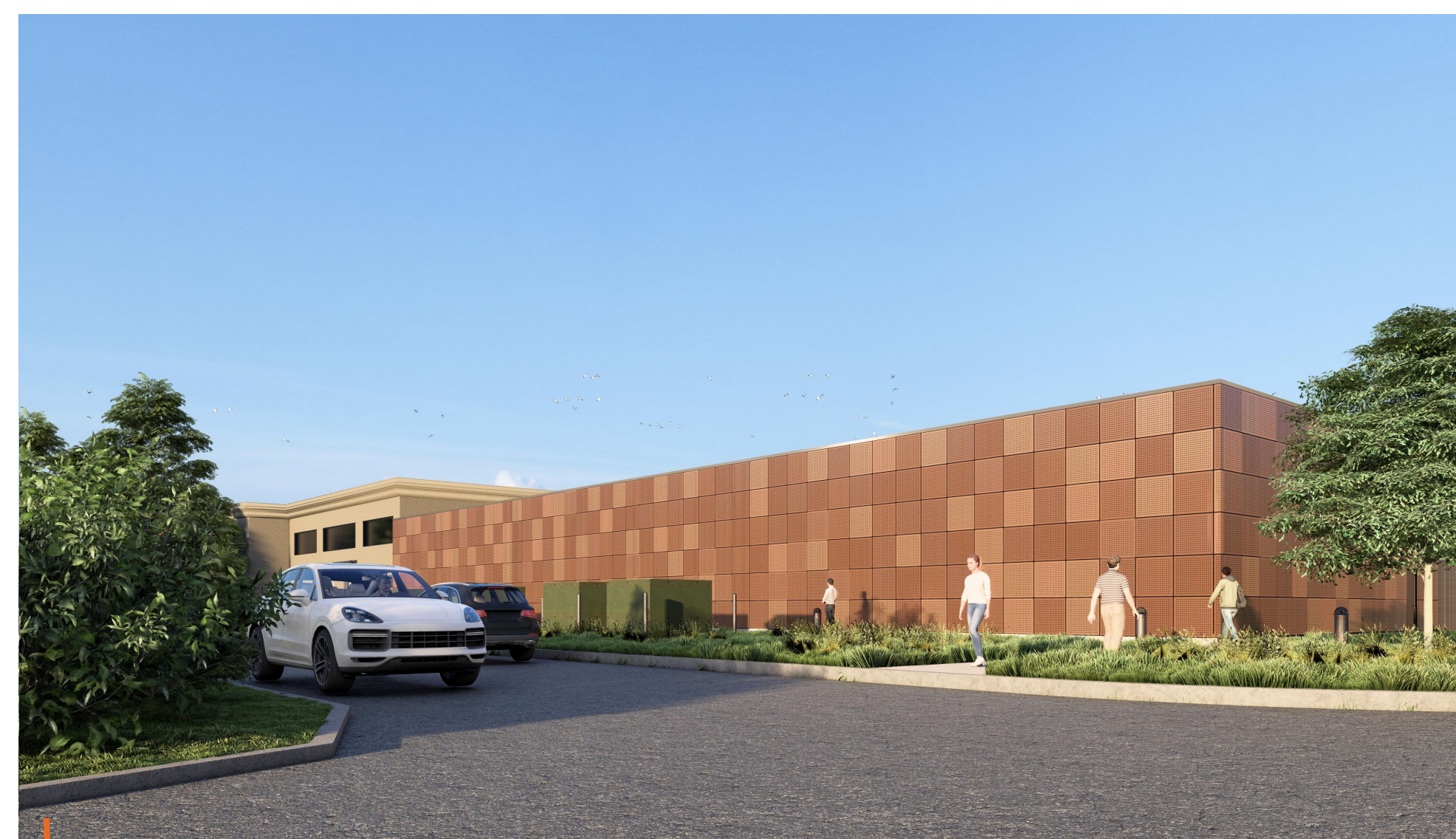
Pedestrian View: The façade consists of a series of perforated metal panels arranged in a uniform grid, creating a modern, textured appearance with subtle geometric patterns. The panels all share a perforated design, but the size and arrangement of the holes vary across panels.
