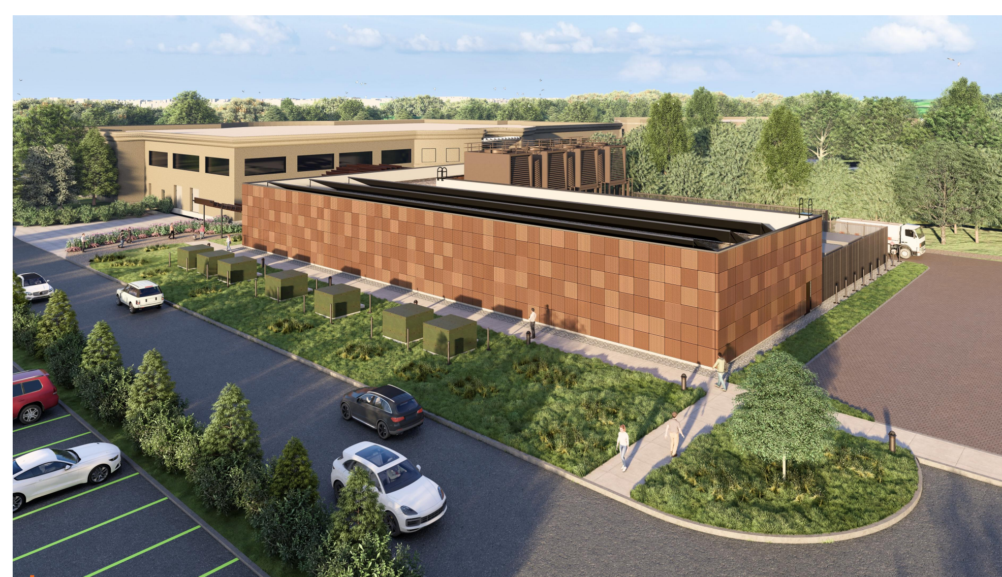
Birds eye view: The design features a modern rectangular building with a patterned perforated rainscreen façade in bronze-like earthy tones, creating a contemporary look. It is set within a landscaped area with greenery, parking spaces, and a wide service driveway for access.
