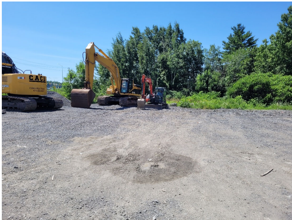
Photograph 6: View of the of the southwest portion of the Phase One Property looking west. View shows construction equipment parking area at the Property.
