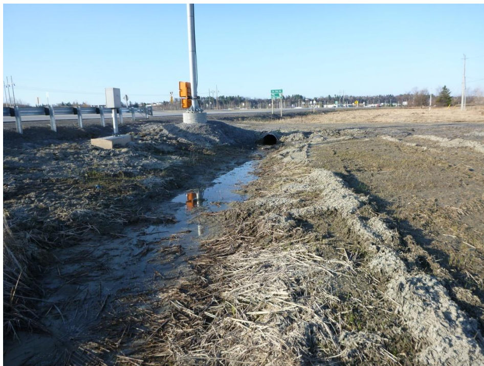
Image 6: Small culvert running parallel to the OR 174, looking south.
