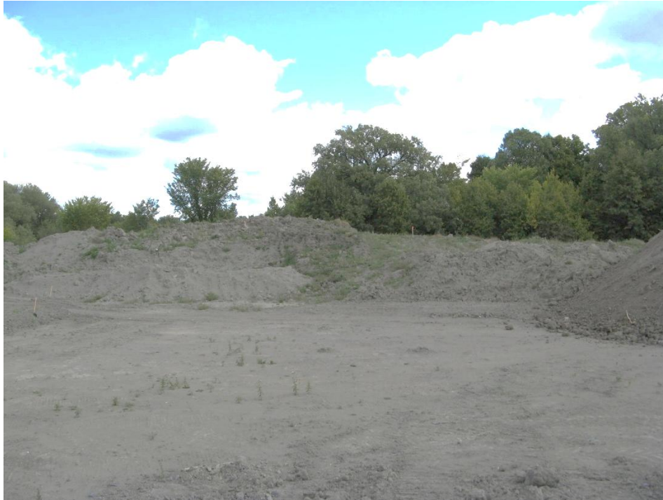
Photo 1 – Current condition of the site. View looking east from Hilversum Lane, with ravine forest edge in the background
