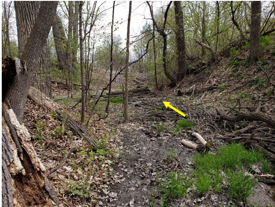
Channel temporarily loses definition before flowing through the second concrete culvert near the downstream extent of the reach.
