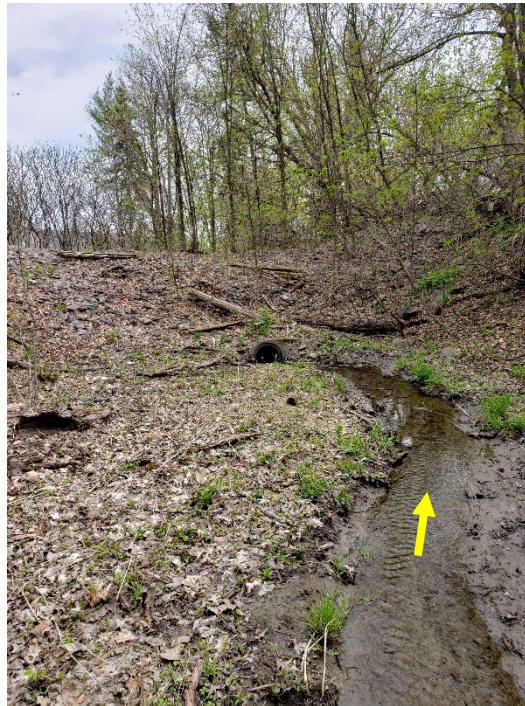
View of the channel as it enters the second concrete culvert.
