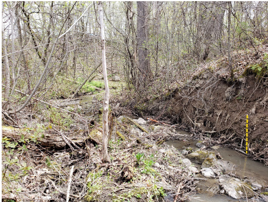
Downstream view with a similar vantage to Photo 19, showing channel adjustment along the valley wall.
