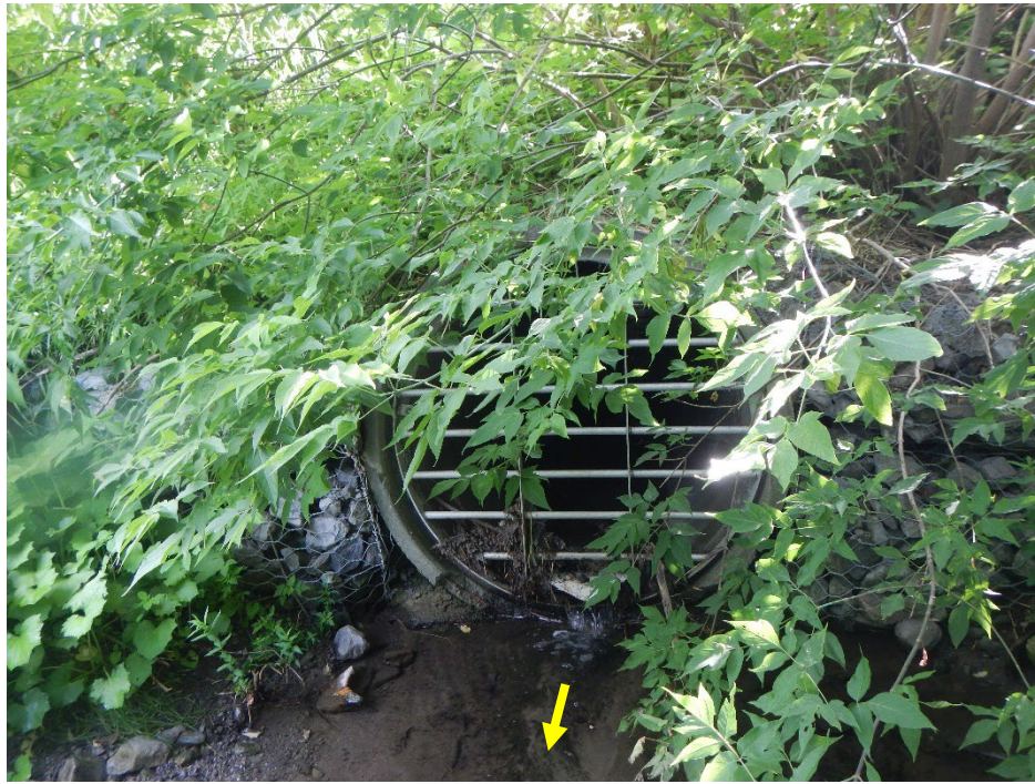
View of the culvert conveying flows under Langstaff Drive.
