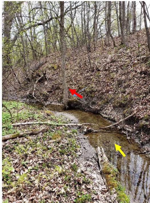
View of a valley wall contact that showed limited channel adjustment at the toe. Note the upright tree at the toe of slope (red arrow).
