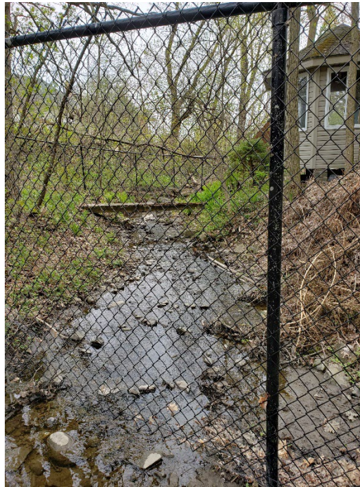
View of the channel downstream, where it flowed through private property.
