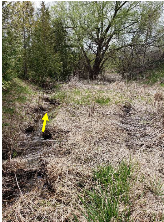
Downstream view of channel where it flowed parallel to the toe of slope.
