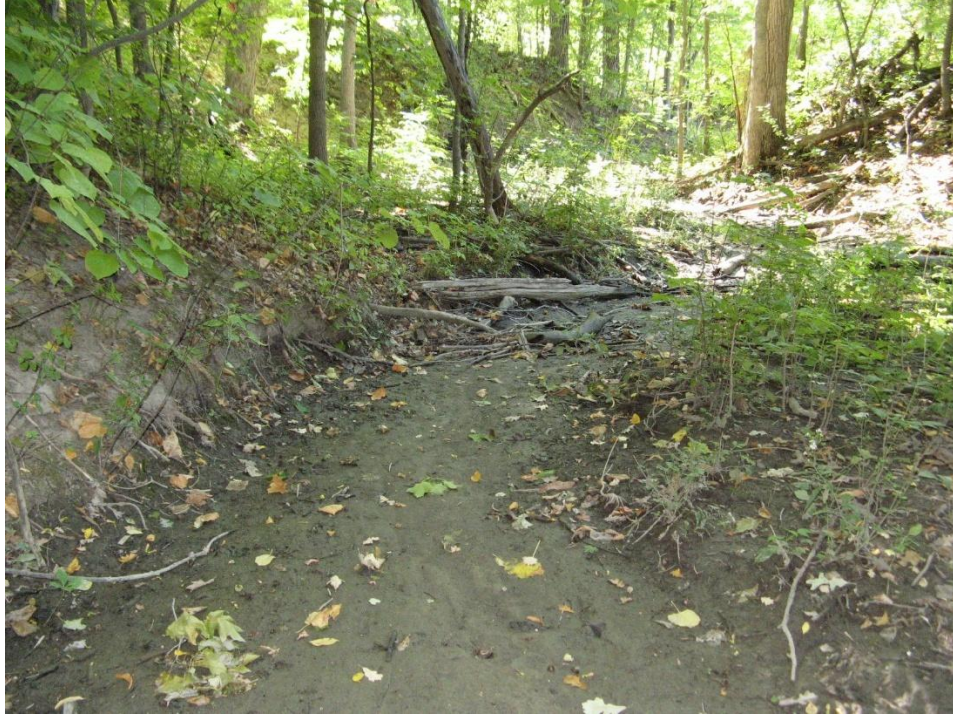
Photo 5 – Channel was dry on September 9 th , 2025 after a very dry August. View looking north
