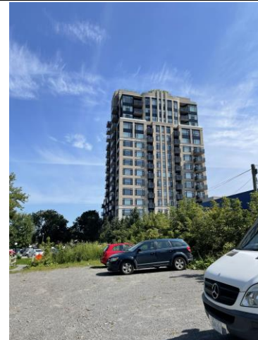
Photo 8 - High rise condominium east of Property. Location of former gas station.
