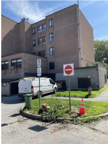
Photo 7 - Unitarian house, adjacent (east) of Phase One Property. Facing east.
