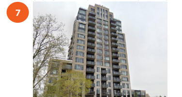
75 CLEARY AVE. 16-STORY RESIDENTIAL BUILDING
