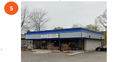
797 RICHMOND RD. EXISTING 1-STORY DENTAL OFFICE
