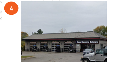
801 RICHMOND RD. EXISTING 1-STORY AUTO SHOP
