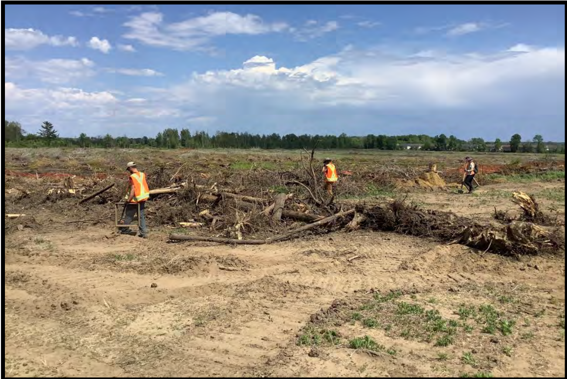
Figure 14: Testing next to tree grubbing south of central wooded area (D78).
