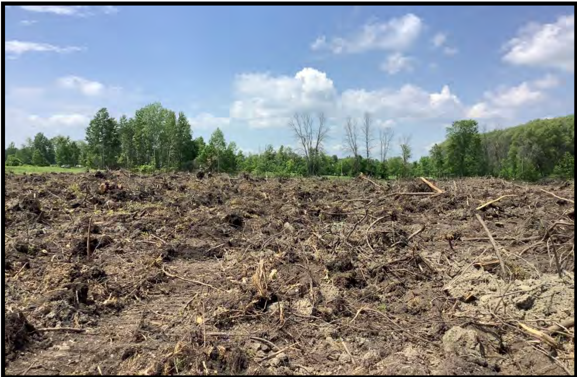
Figure 8: grubbed trees and disturbed soils, showing exposed subsoil (D113).
