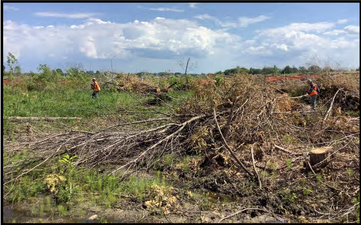
Figure 33: Testing through grubbed trees in southern study area (D80).
