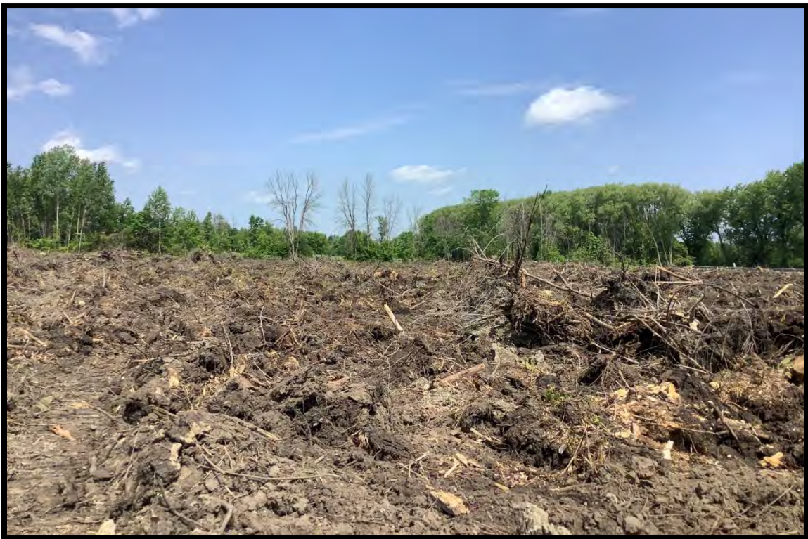
Figure 6: grubbed trees and disturbed soils, showing exposed subsoil (D111).
