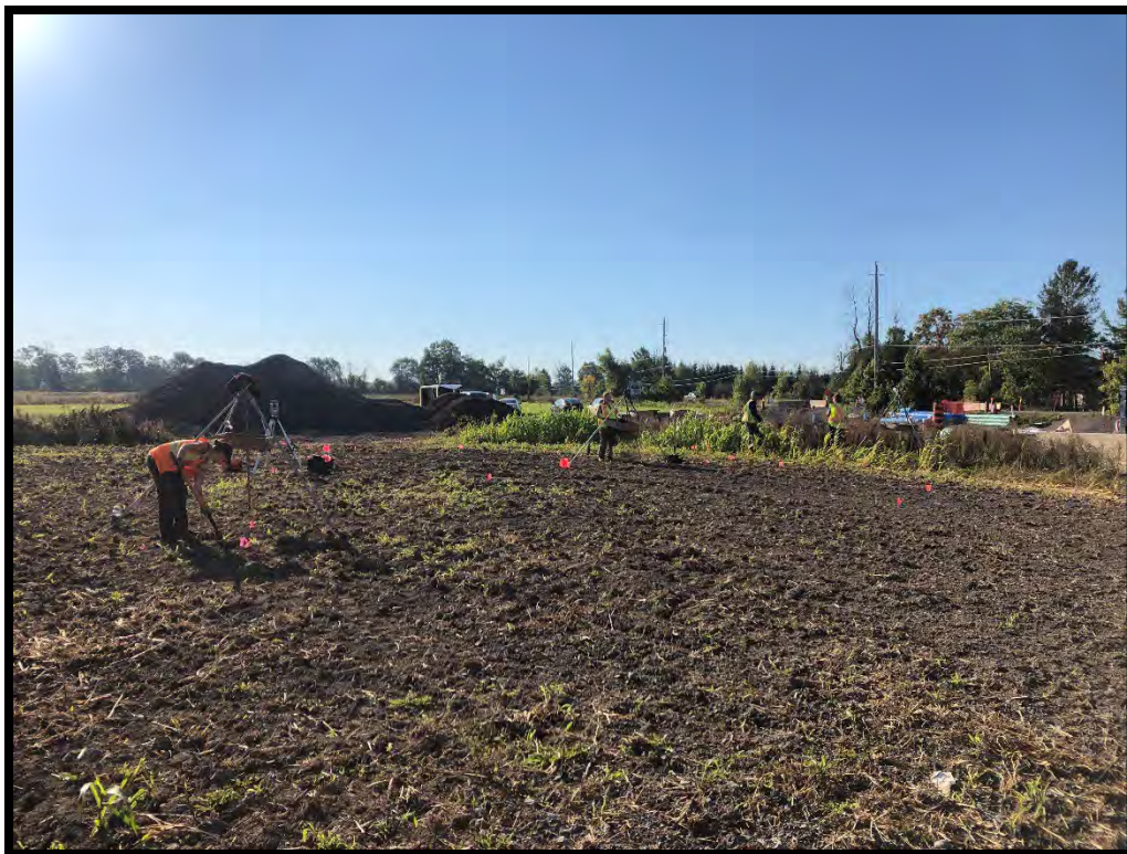
Figure 16: Completing CSP, setting up grid, and commencing excavation (MH1037-D004).
