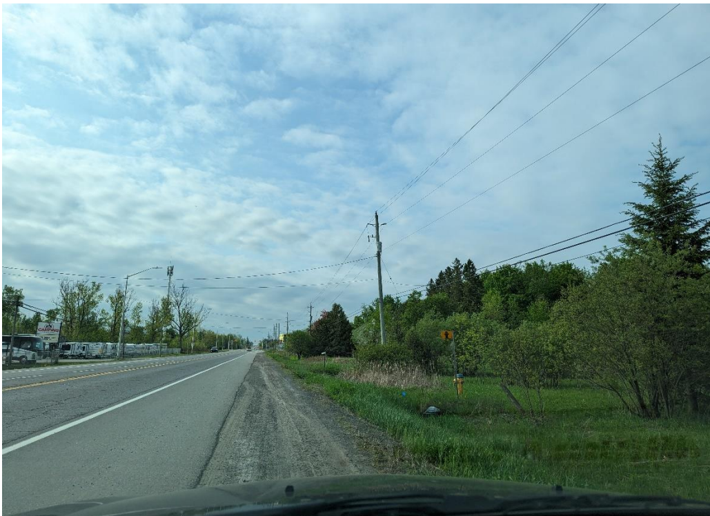
Photograph 8: View looking south, along the west side of Bank Street towards 4820 Bank Street – PCA 3 (pole mounted transformer).
