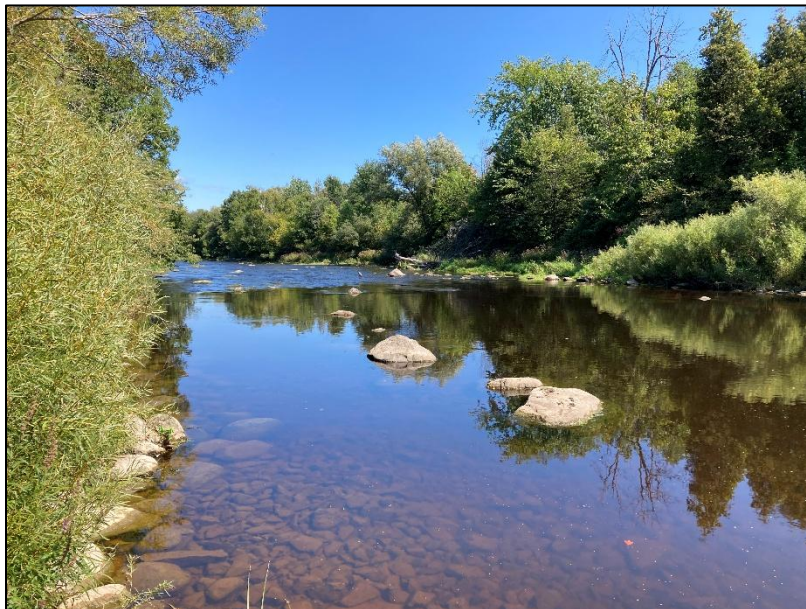
Photo 4: Observed riprap at the toe of the slope along the full property frontage adjacent to the river. In addition, the slope face was observed to be covered by mature vegetation and small trees. No evidence of active erosion was observed along the toe of the slope – facing northeast.
