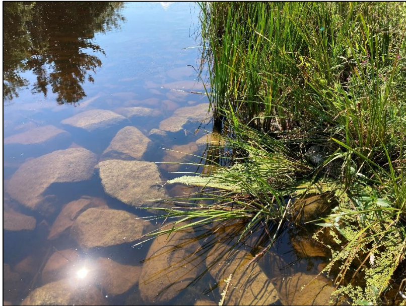
Photo 4: Observed riprap at the toe of the slope along the full property frontage adjacent to the river. In addition, the slope face was observed to be covered by mature vegetation and small trees. No evidence of active erosion was observed along the toe of the slope – facing northeast.
