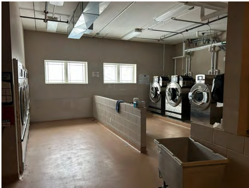
Photo 10 View of the staff laundry room located on the first level of the Site building.
