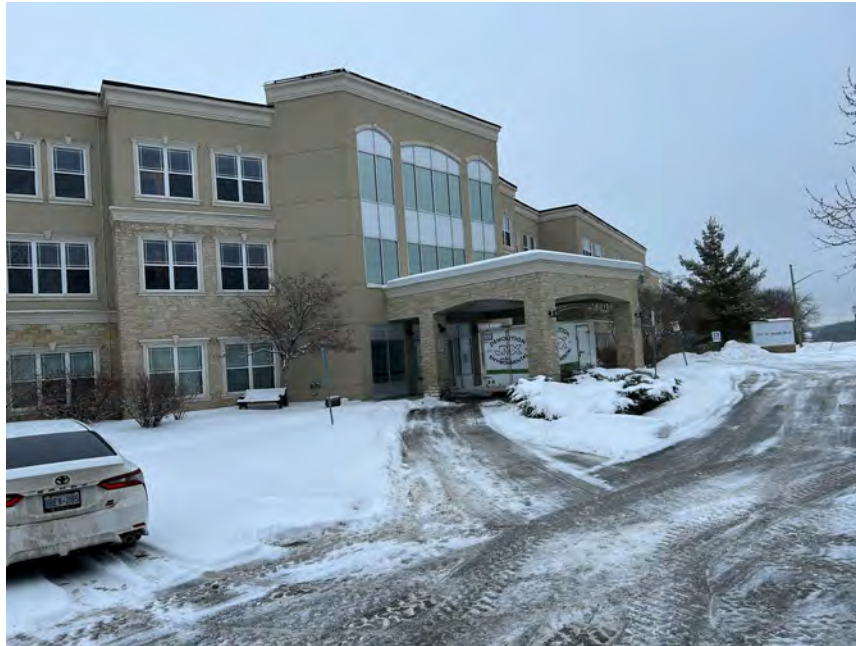
Photo 1 View of the southern portion of the Site building, facing northeast.
