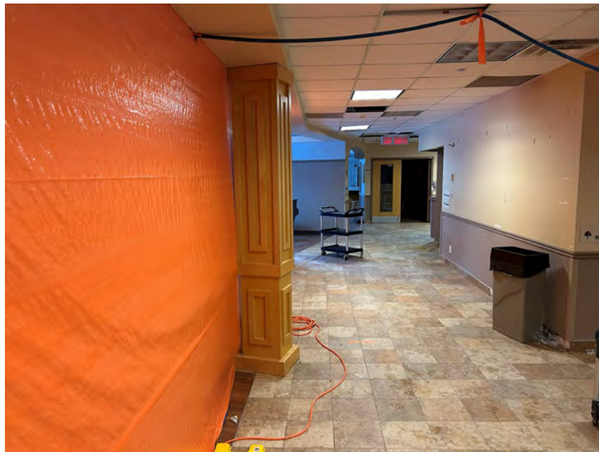
Photo 2 Photo showing the reception area of the Site building.
