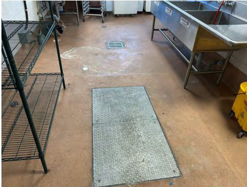
Photo 9 Photo showing the grease trap located in the kitchen of the Site building.
