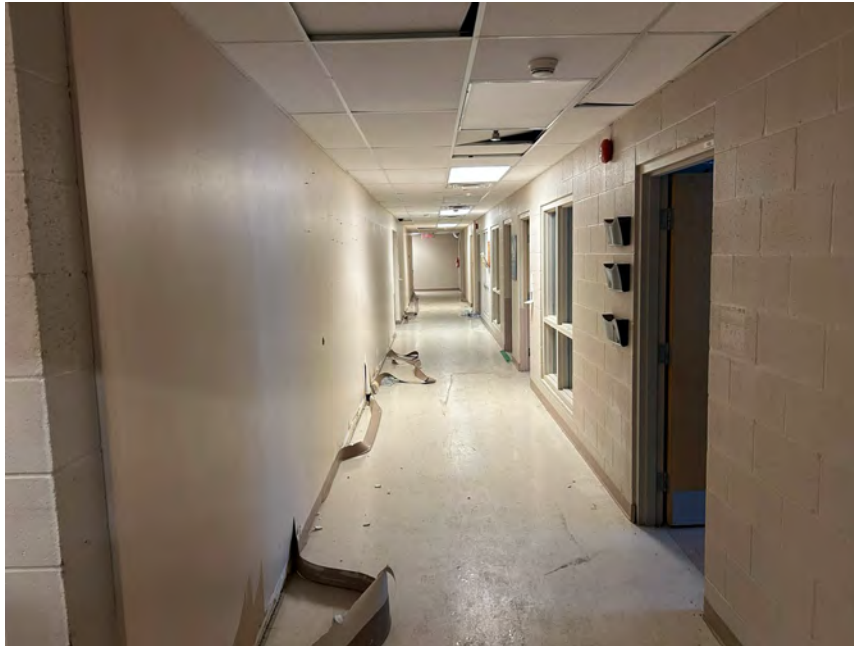
Photo 5 View of a typical hallway in the Site building.
