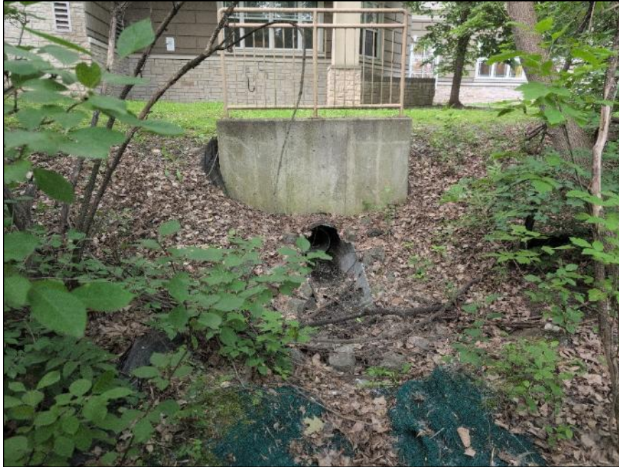
Image 11: Culvert near the northern property limit.
