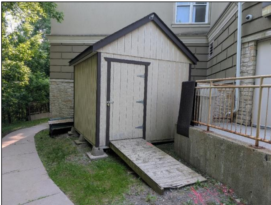
Image 6: Storage shed and walkway at the top of bank. Note red paint indicating buried utilities.
