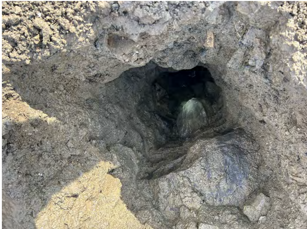
Photo 7 - View of test pit TP-05
