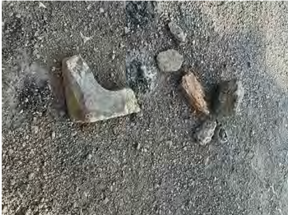
Photo 6 - View of construction debris observed in TP-04
