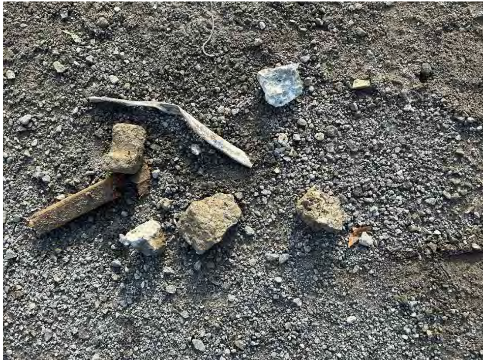
Photo 3 - View of construction debris observed in TP-02
