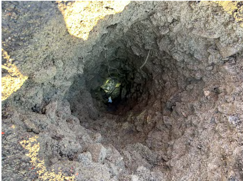
Photo 10 - View of test pit TP-08
