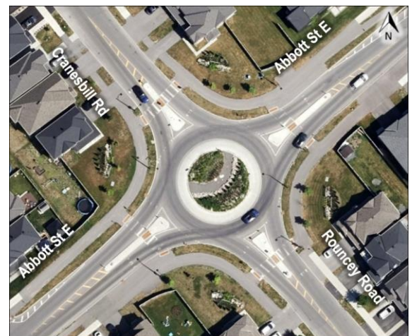
Figure 4: Abbott Street East at Cranesbill Road / Rouncey Road
