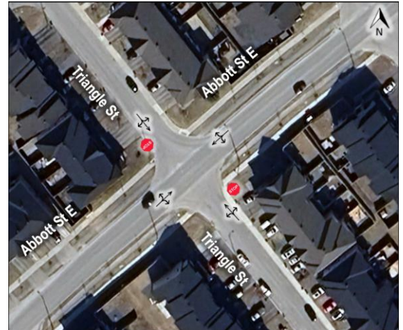
Figure 5: Abbott Street East at Cranesbill Road / Rouncey Road
