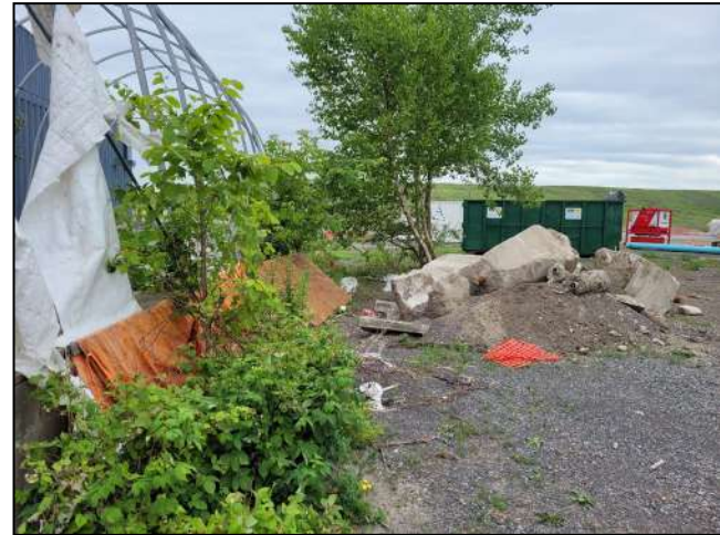
Photo 6: Exterior view of shed, note debris and vegetation (Photo taken looking south).
