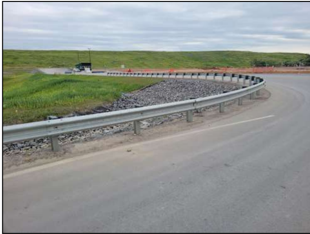
Photo 17: Weigh scale and surface water pond, southeast of site (Photo taken looking southwest).
