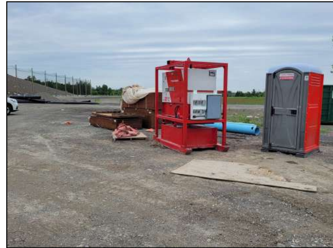
Photo 10: View of on-site storage (Photo taken looking northwest).
