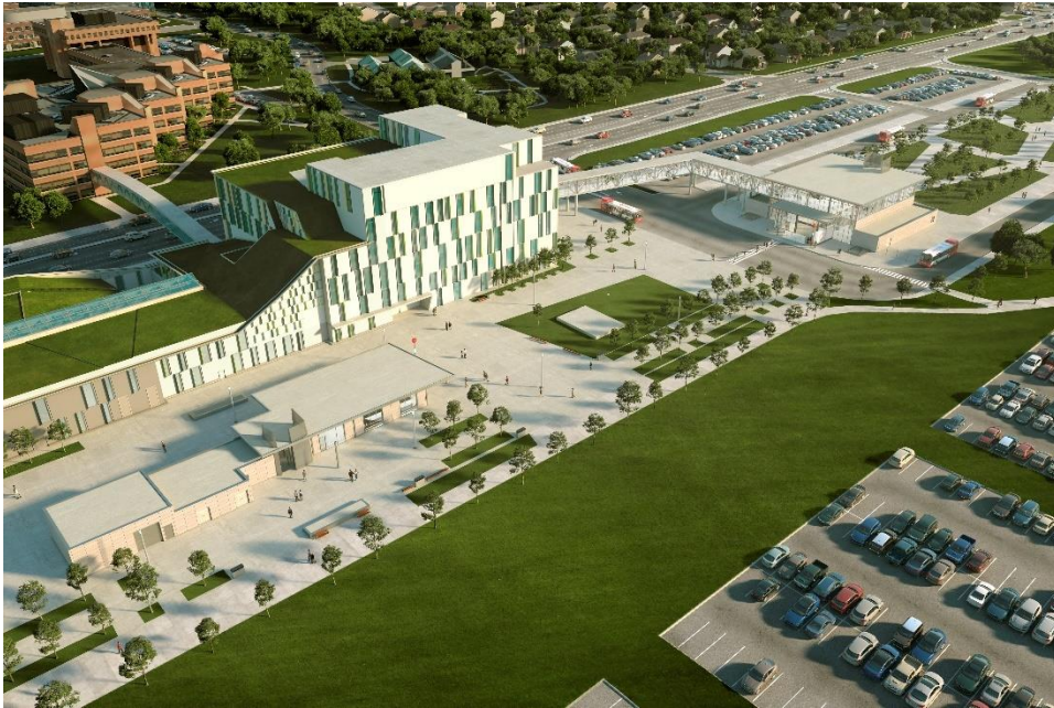
Figure 2-13: Future Algonquin Station
