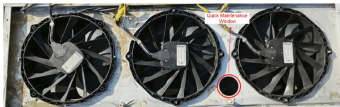
figure 5-36 Schematic Diagram of Quick Maintenance Window
