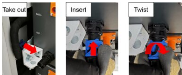
figure 5-26 Installation of Bidirectional Shut-off Valve (Left Side)
