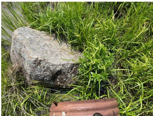
Photo 12 Facing down at existing conditions of Reach 2 and metal culvert, June 3, 2025.
