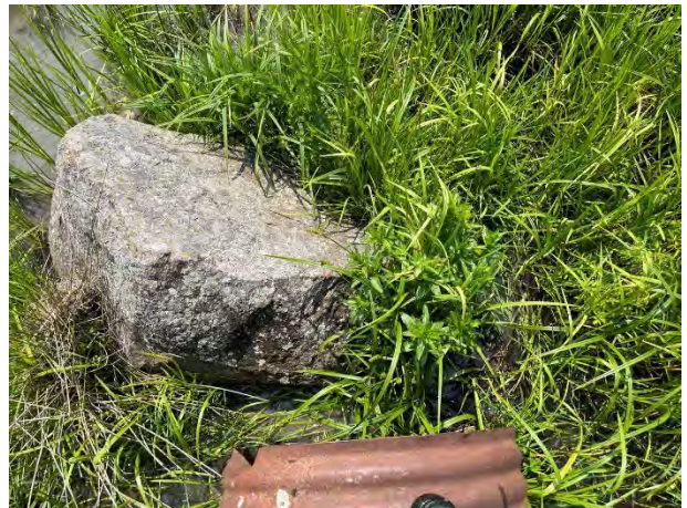
Photo 12: Facing down at existing conditions of Reach 2 and metal culvert, June 3 2025.
