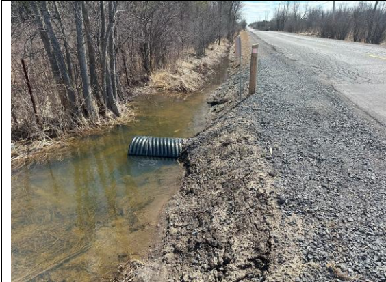
Photo 27: Side view at location S18 (Figure 3-1) on April 7, 2025.
