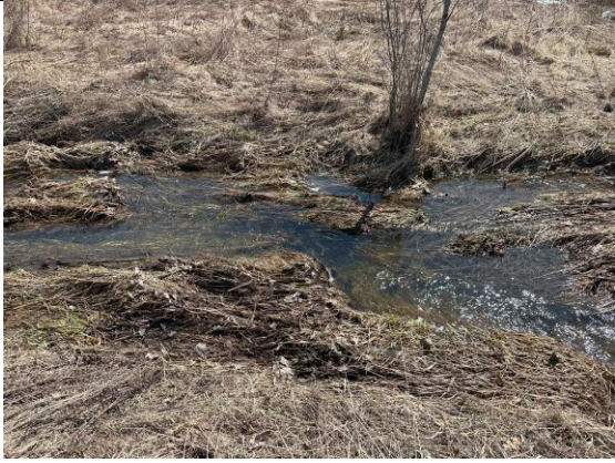
Photo 23: Side view at location S16 (Figure 3-1) on April 7, 2025.
