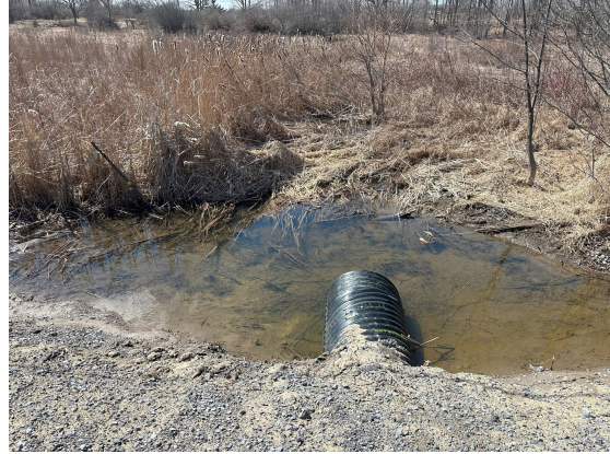
Photo 26: View looking southwest (Upstream) at location S18 (Figure 3-1) on April 7, 2025.
