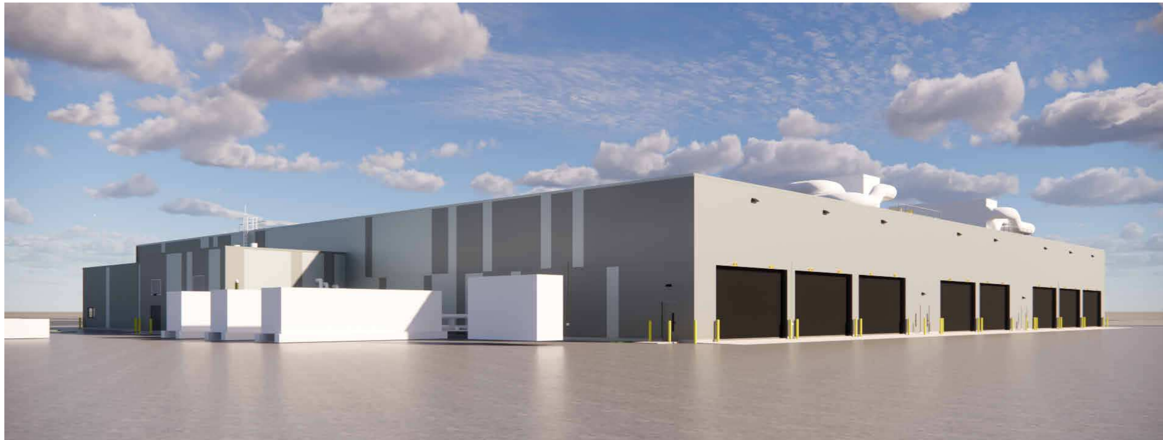
VIEW OF THE BUILDING APPROACHING NORTH-WEST CORNER
