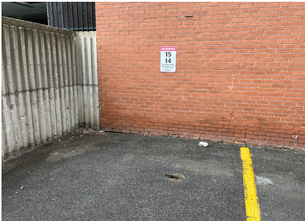
Photograph 6: Location of existing monitoring well at the rear of the parking lot.
