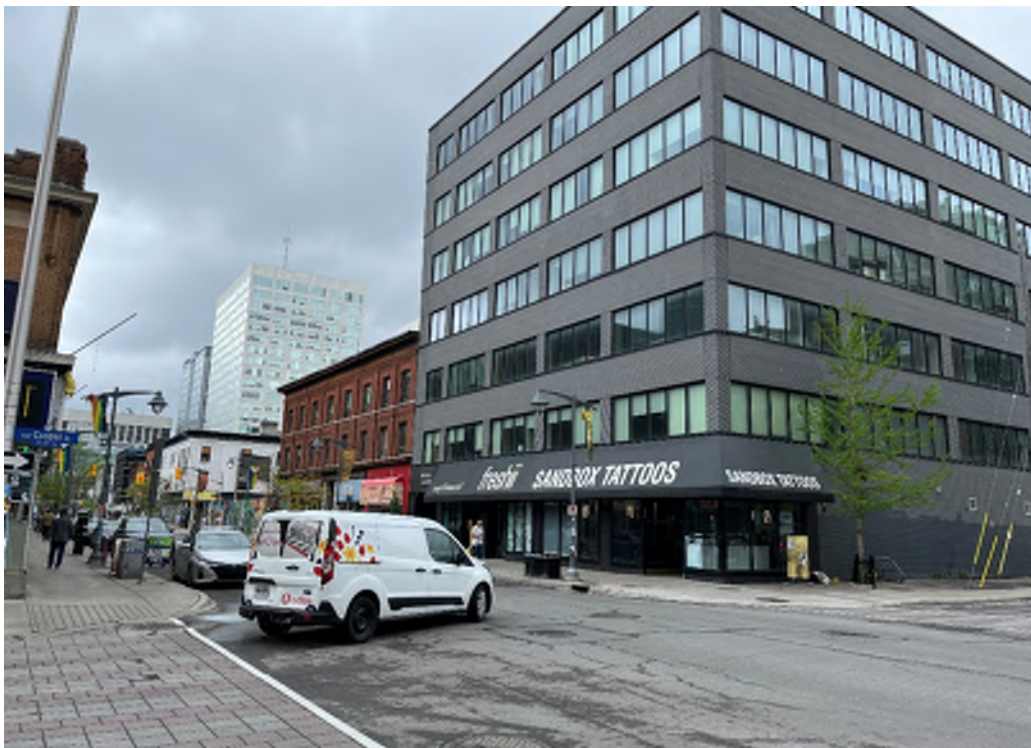
Photograph 4: View to the north down Bank Street
