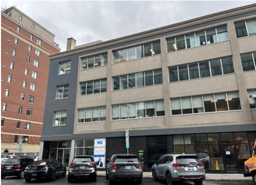
Photograph 3: View of the subject building, looking south from Cooper Street.
