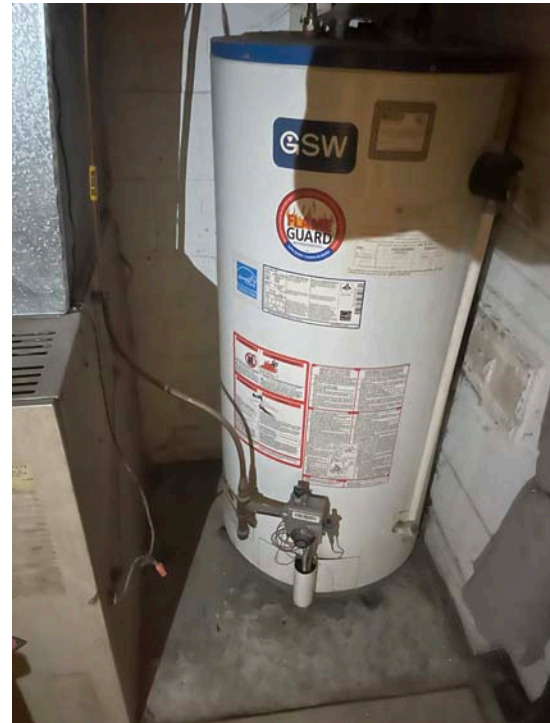
Example of natural gas powered furnace and water heater at 342/344 Queen Mary Street
