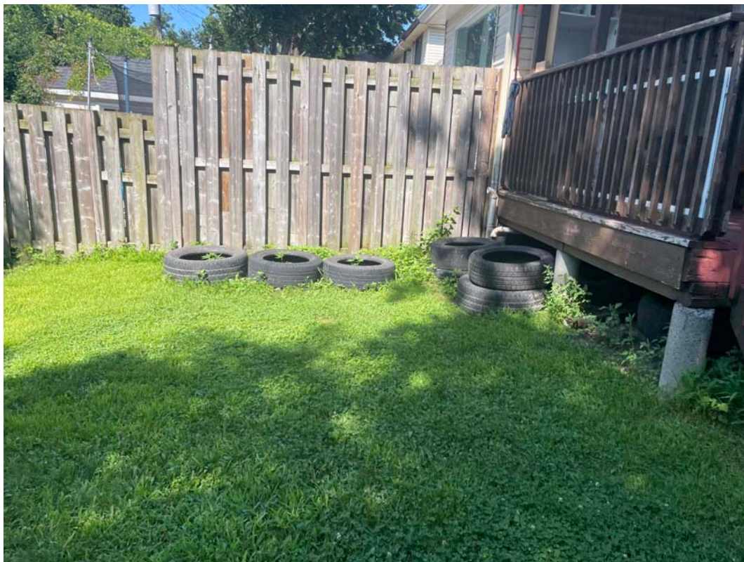
Rear view of 348/350 Queen Mary Street
