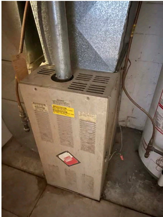
Example of natural gas powered furnace and water heater at 342/344 Queen Mary Street
