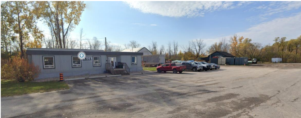
Figure 7: Portable office and parking, looking south
