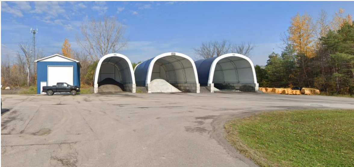
Figure 5: Existing structure on the subject site, looking north
