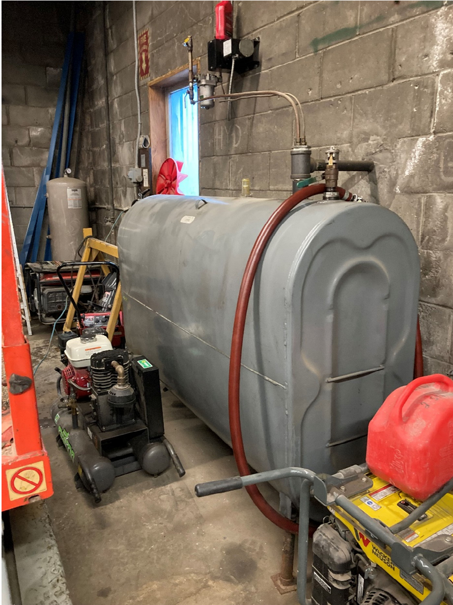
Photograph 11: Double walled 1000L steel shop tank from 1994 containing furnace oil.
