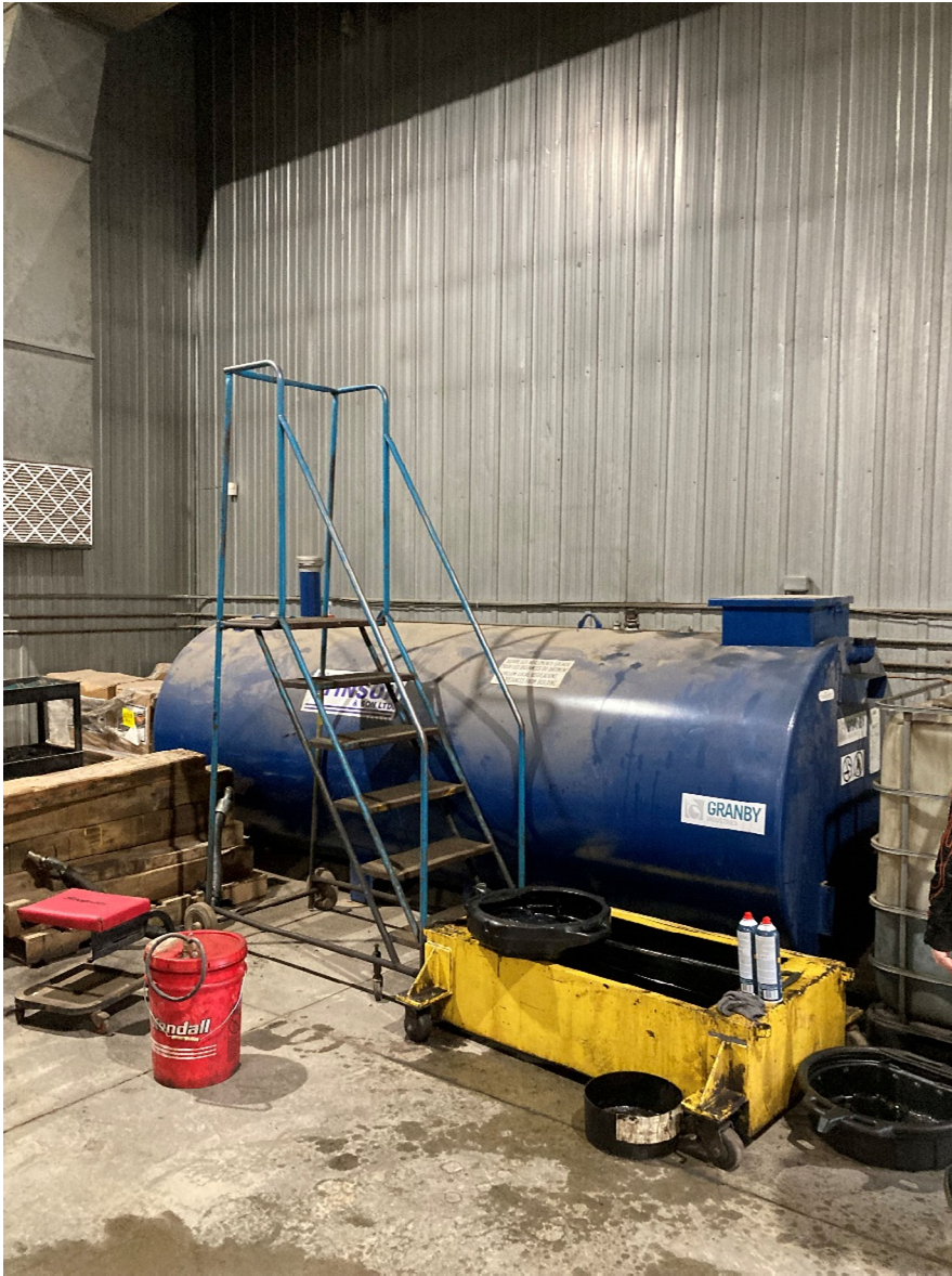
Photograph 9: Fuel storage tank from 2021 containing 1000L of waste oil
