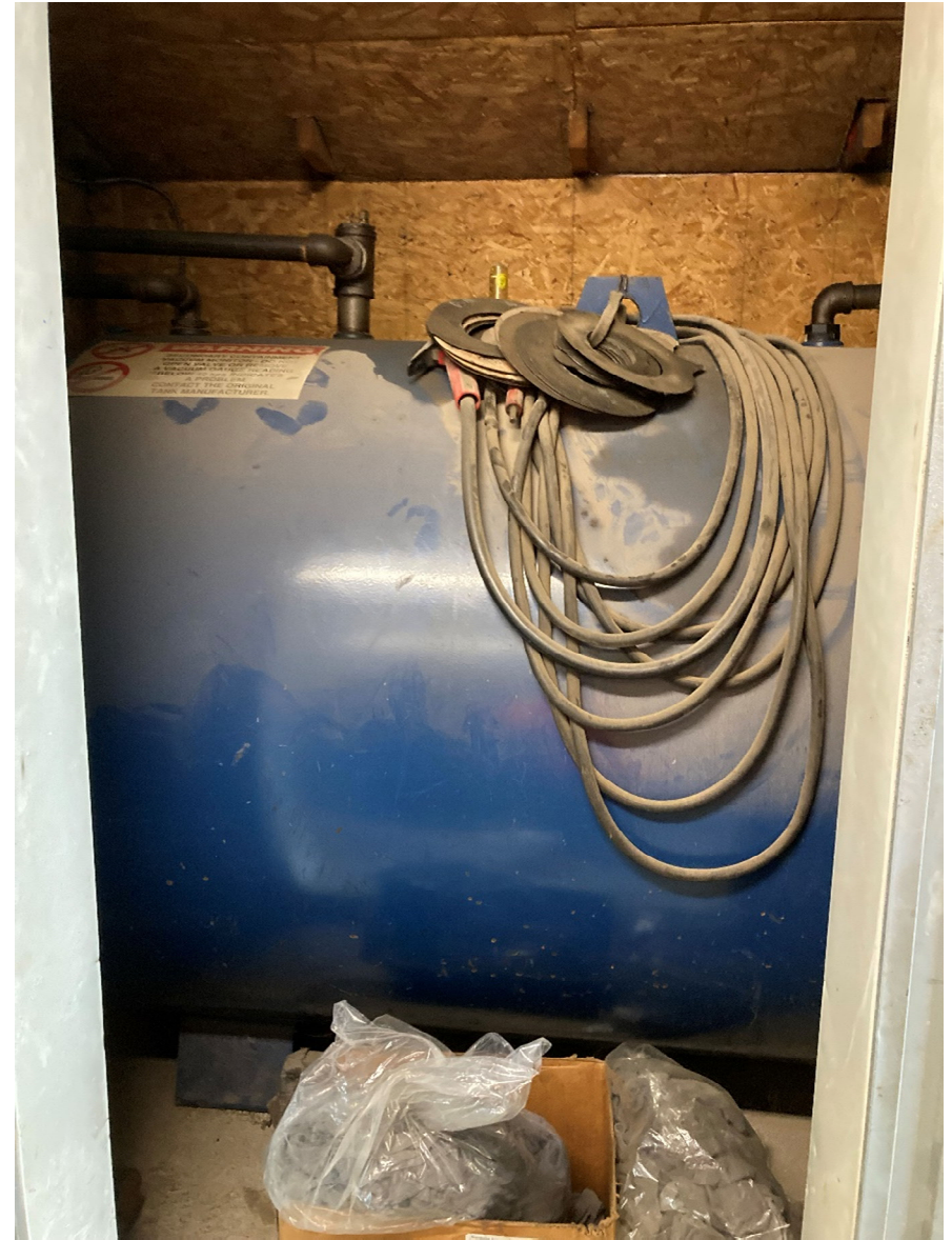
Photograph 10: Interior furnace oil tank containing 1000 L of furnace oil.
