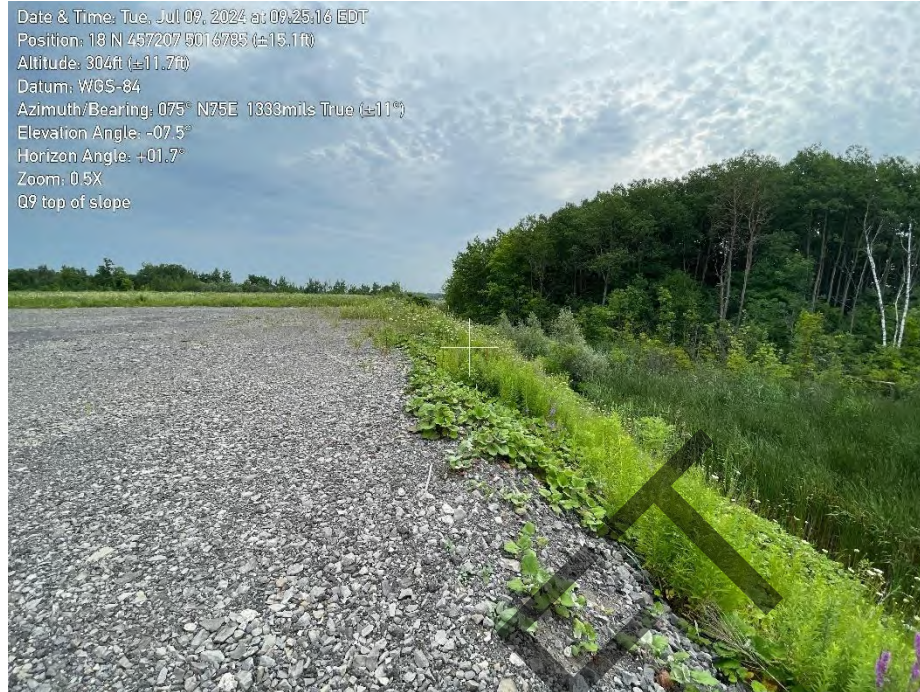
Figure 4 Top of slope, looking east
