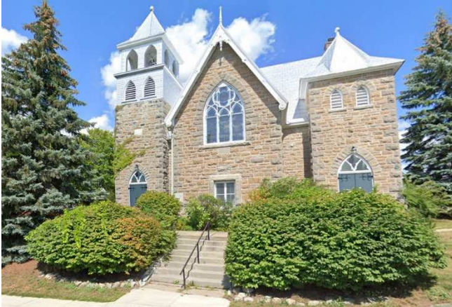
Figure 19. Heritage Overlay Designated Property, 5567 Manotick Main St. (Manotick United Church)
