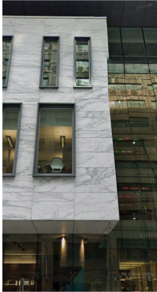
Masonry volume bisected by curtain wall
