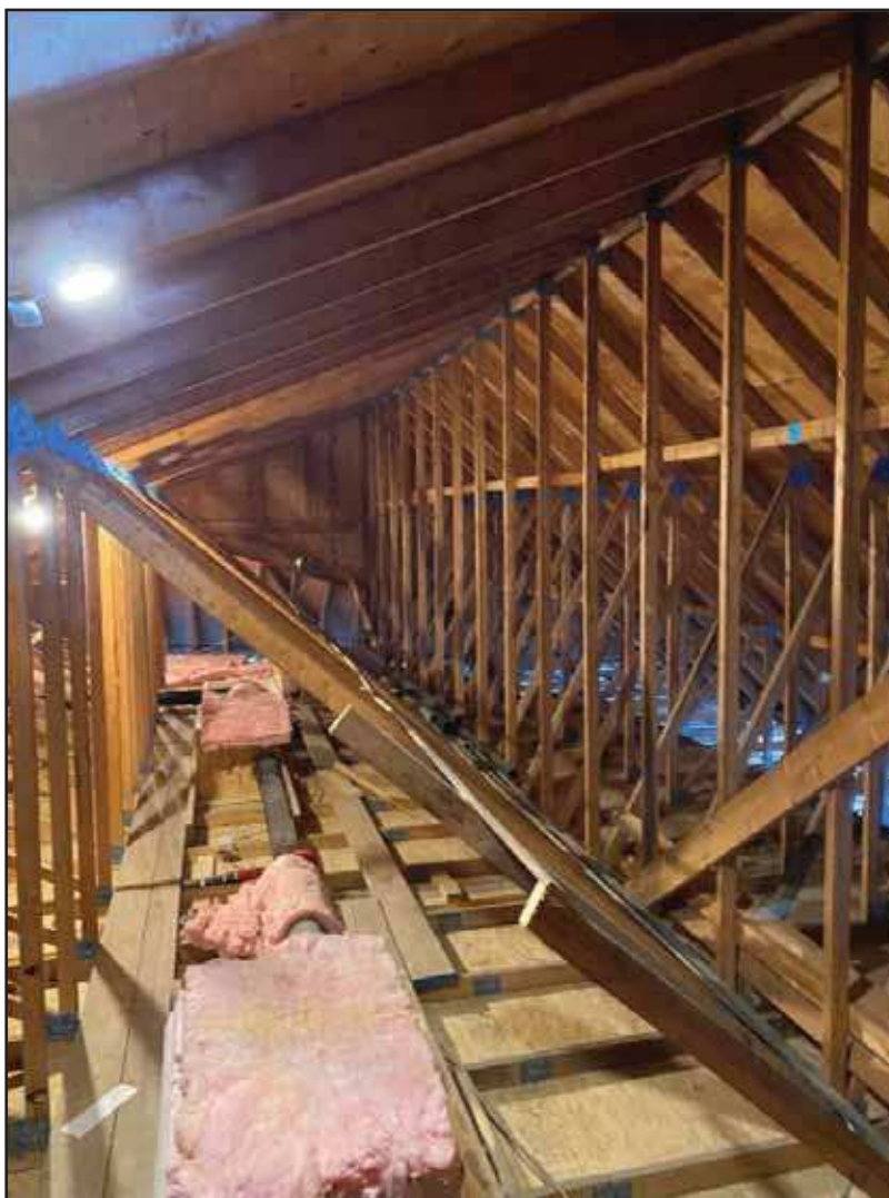
Photograph 14: View of attic above car wash.
