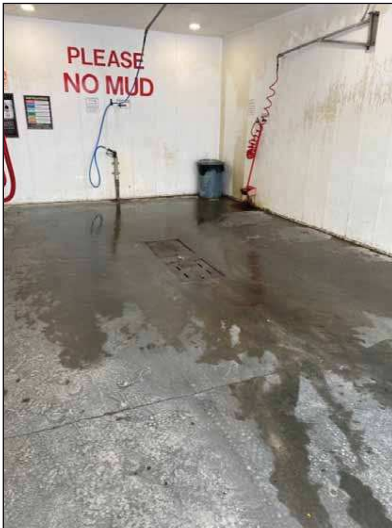
Photograph 9: Interior view of a car wash bay.
