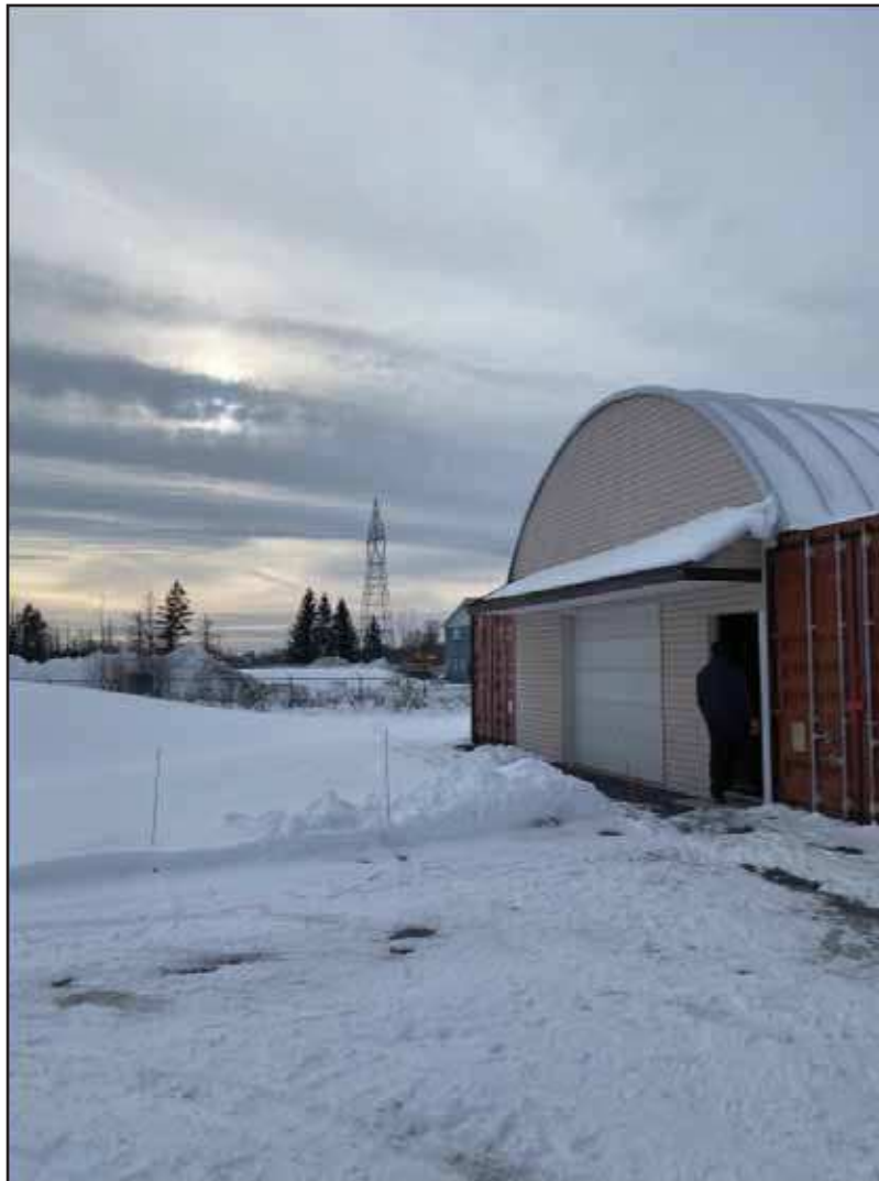
Photograph 6: View of the recently build storage building.
