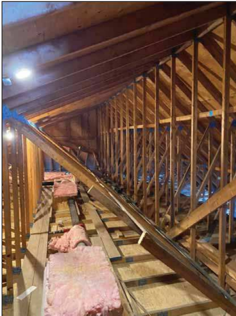
Photograph 14: View of attic above car wash.
