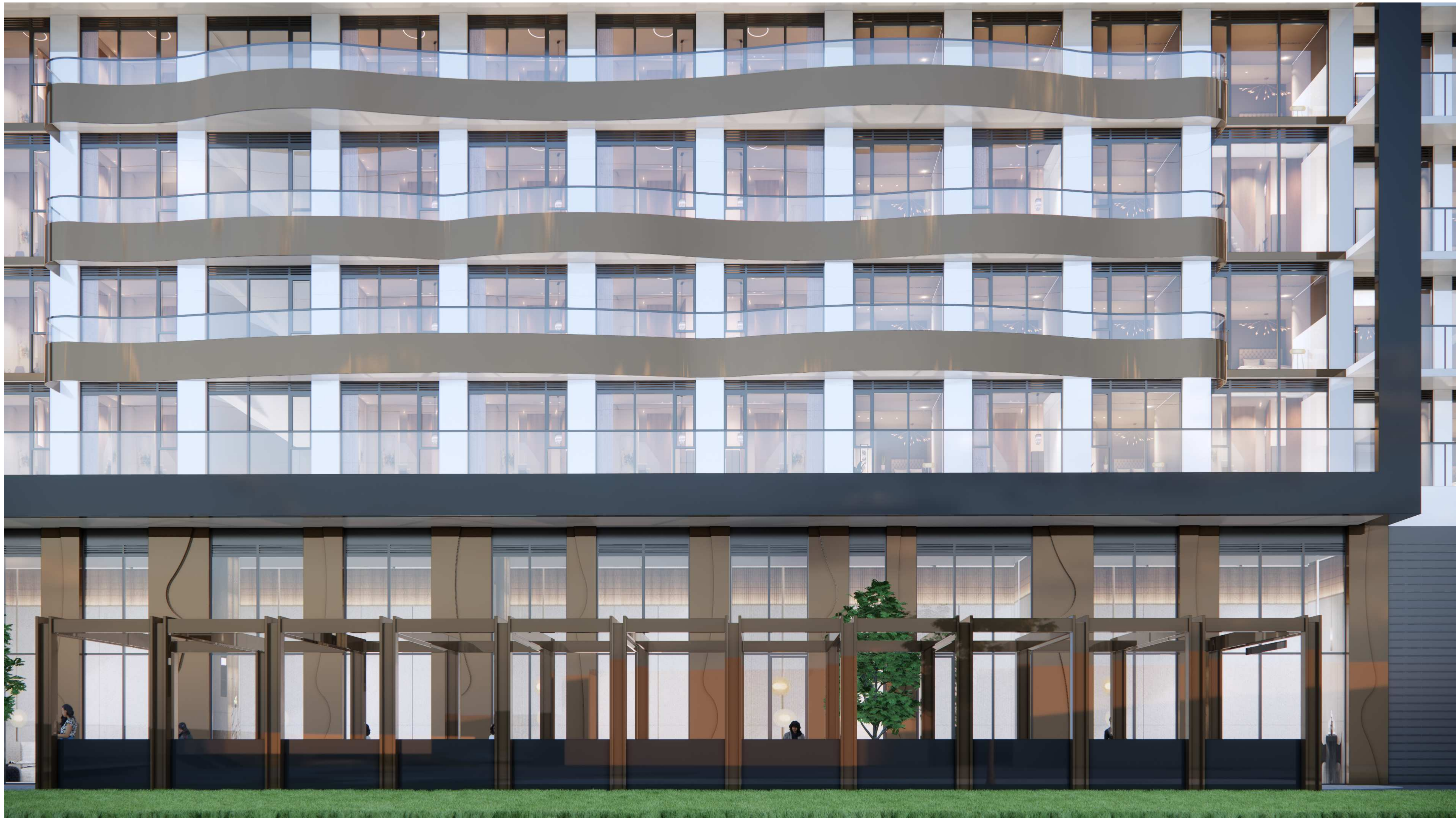
VIEW LOOKING WEST TOWARDS THE PARKING RAMP TRELLIS STRUCTURE
