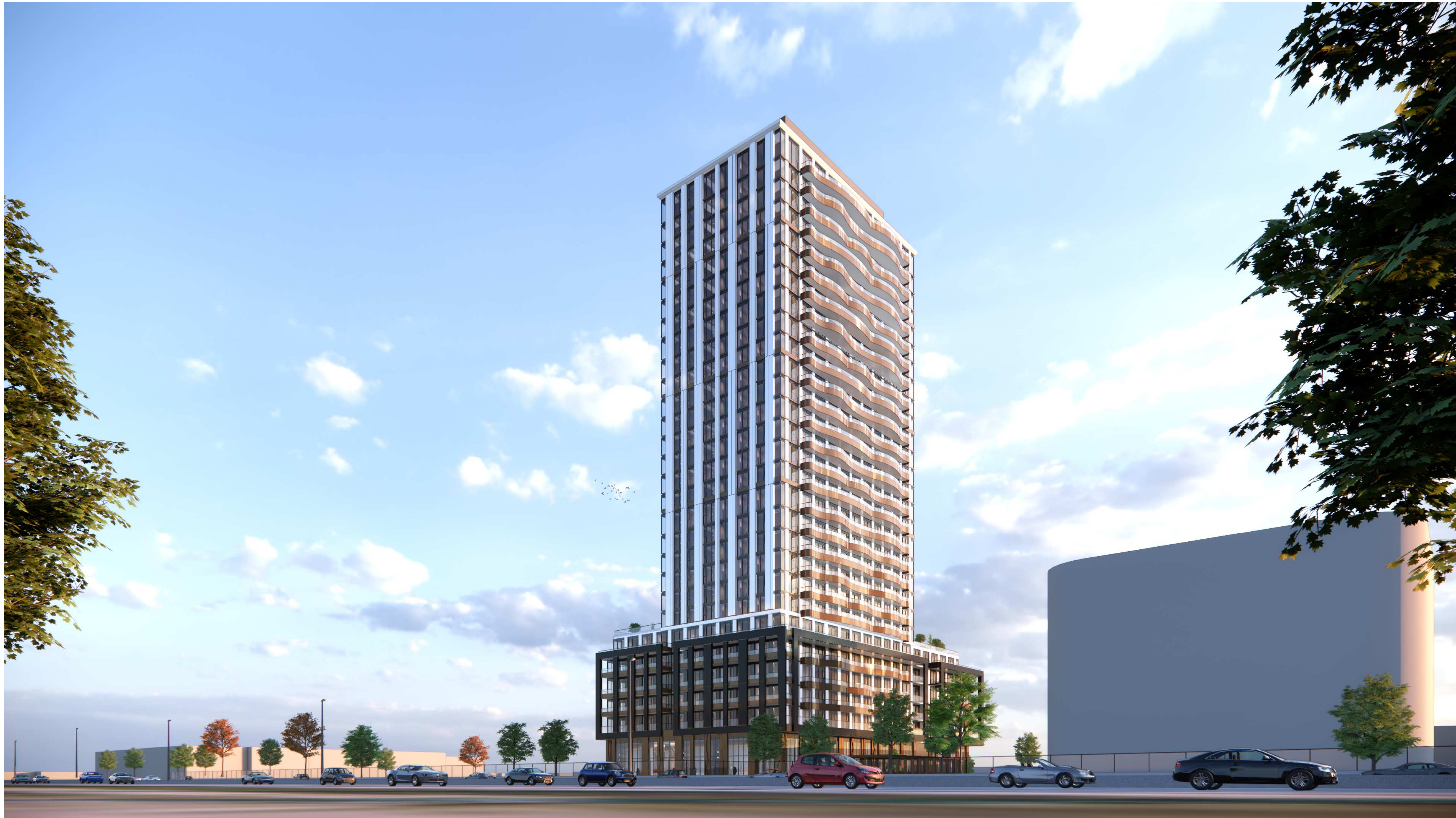
VIEW FROM TRANS-CANADA HWY LOOKING NORTH WEST
