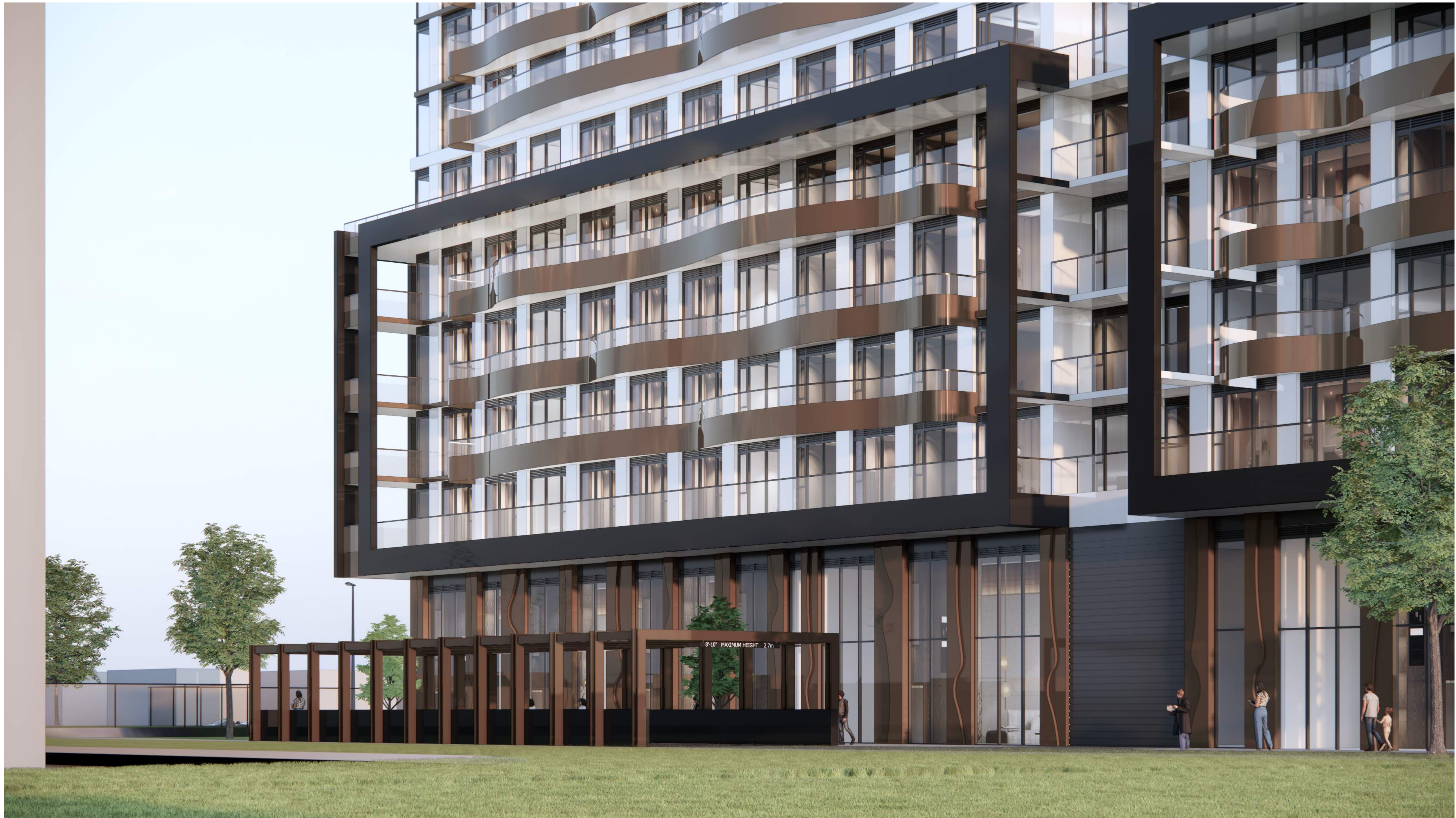
VIEW LOOKING SOUTH WEST TOWARDS THE PARKING RAMP TRELLIS STRUCTURE
