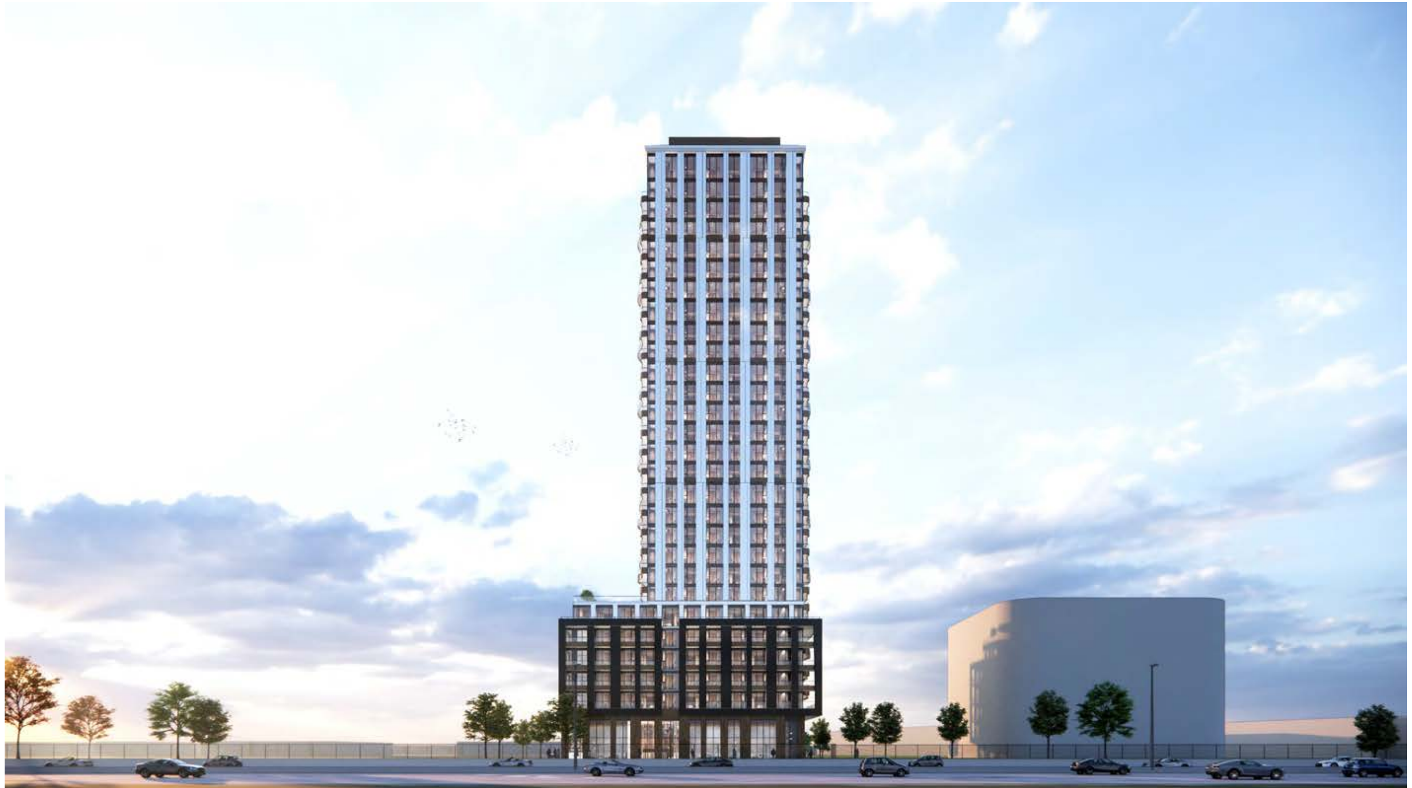
VIEW FROM TRANS-CANADA HWY LOOKING TOWARDS NORTH
