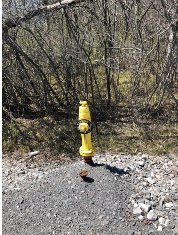
Photograph 10. View of low-lying wet area behind hydrant from road. Note elevation difference.
