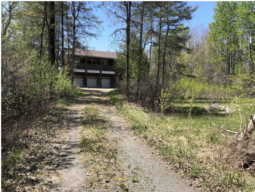
Photograph 9: Property #5494. View of house and associated landscaping. To the left, slopes down to a low-lying wet area. To the right – fill.
