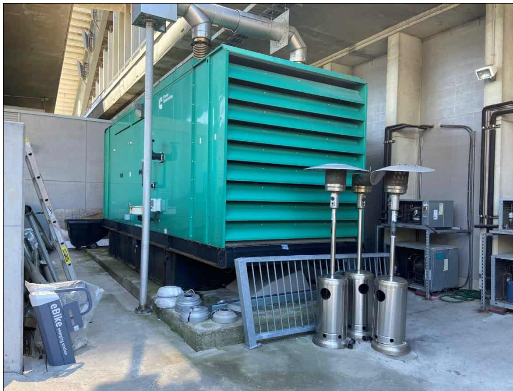
Photo 12: Back-up generator located outside the loading dock area on the east side of TD Place Stadium. Fitted with a 5,791 L capacity diesel storage tank. Date: 06/28/24 Direction: South
