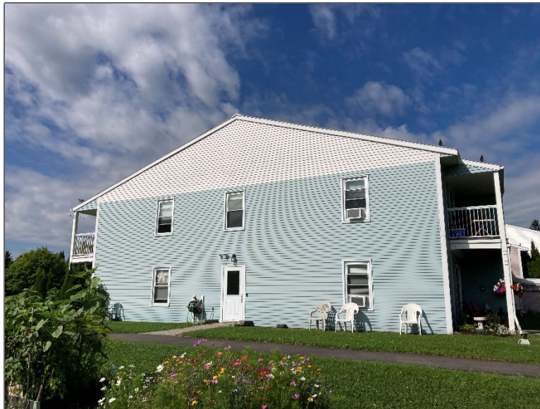
Photo 2 – Site Building (east elevation).
