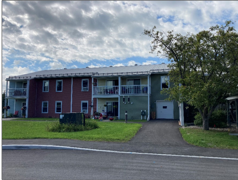
Photo 1 – Site Building (north elevation).
