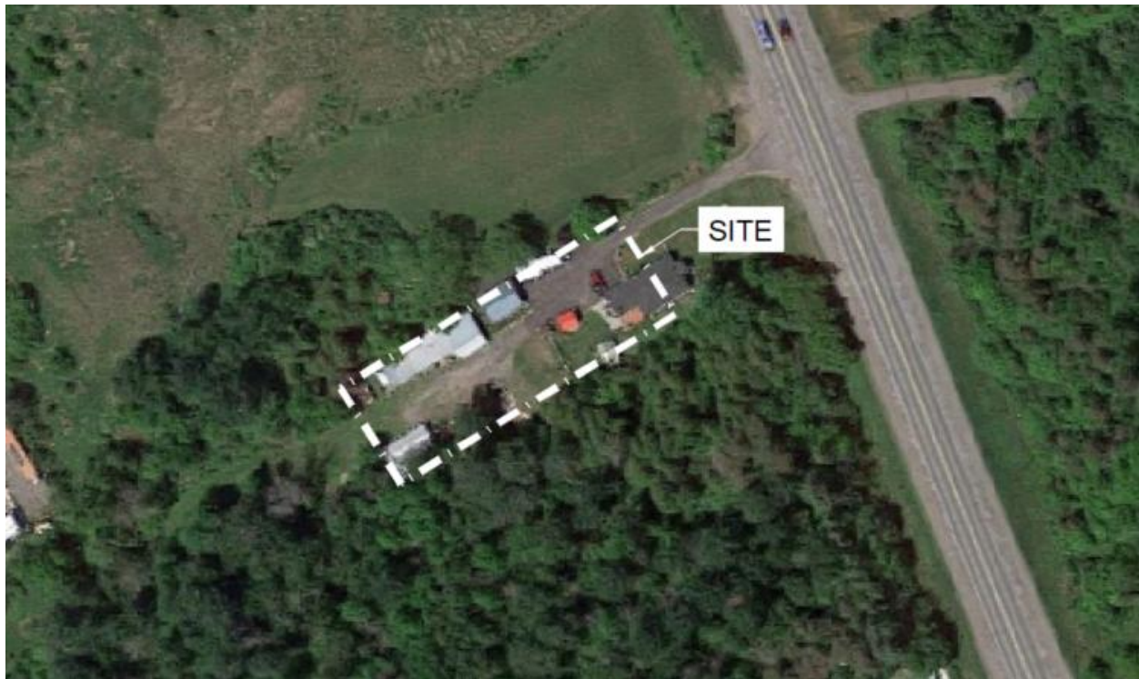
Figure 1: Aerial View of Proposed Development
